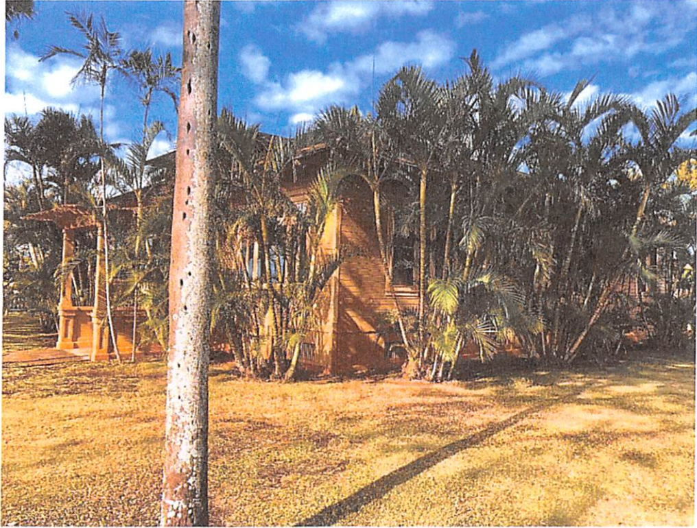
Photo C: View of Museum Building Looking West
