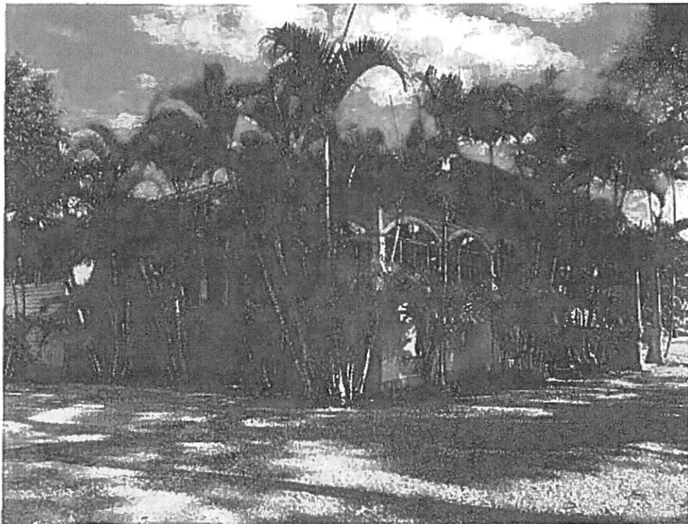
Photo B: View of Museum Building Looking North
