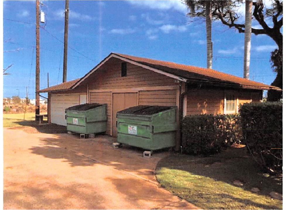
Photo No. 4: View of Garage and Maintenance Shed
