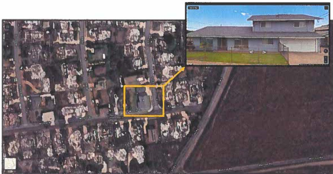
Figure 4: An example of a home that survive, with low density fuel coverage, especially in the 0-5-foot home ignition zone, an asphalt shingle roof, and non- combustible concrete masonry unit wall material. Post-fire imagery courtesy of Maxar and pre-fire condition image courtesy of Google-Street View.
