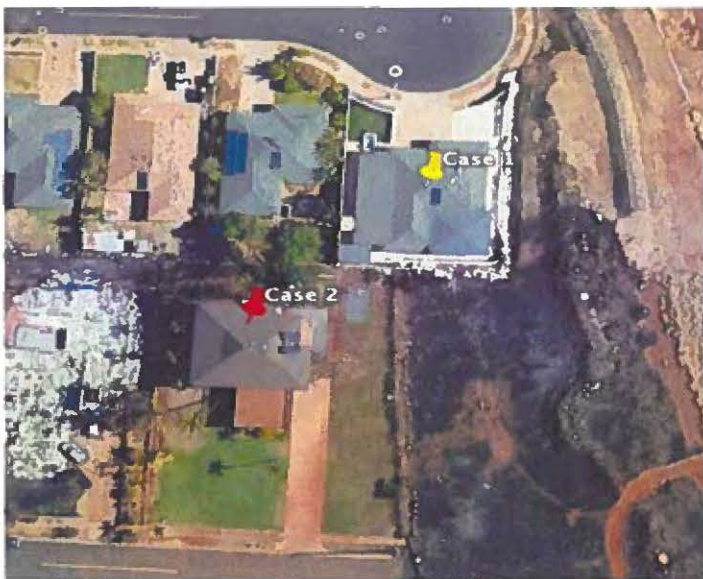
Figure 3. Homes in northern Lahaina that did not burn because of disconnected fuel as the fire propagated from the wildland on the right side of the image.
