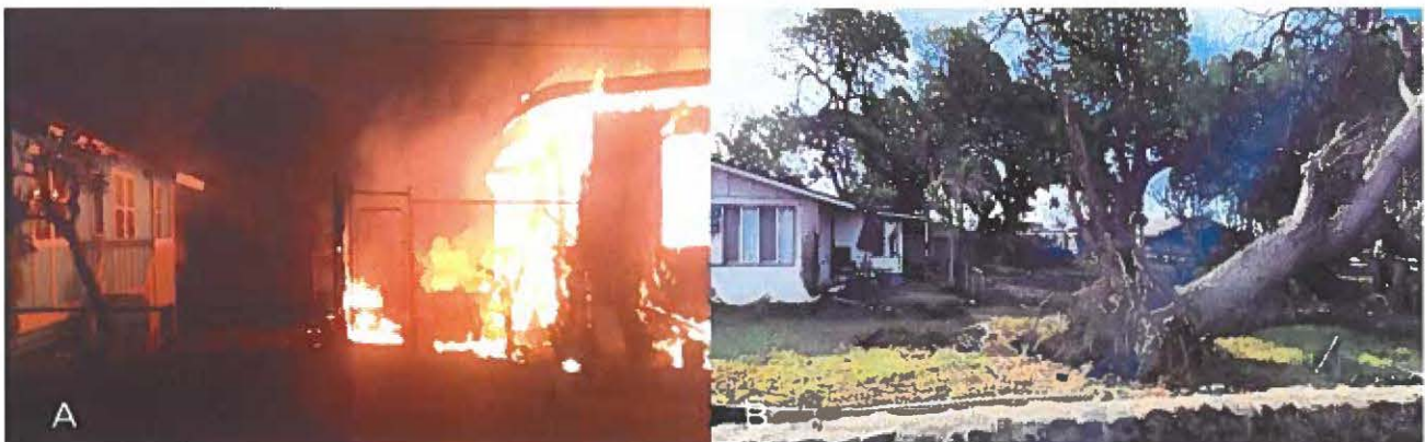
Figure 5. Examples of reduced exposure with non-connective fuel (A) The building on the left of image experienced minor damage due to radiation only (no connective fuel). (B) Embers ignited the combustible fence and vegetation on the leeward side of this building, leading to minor damage. The attached combustible fence was likely disconnected during the event.
