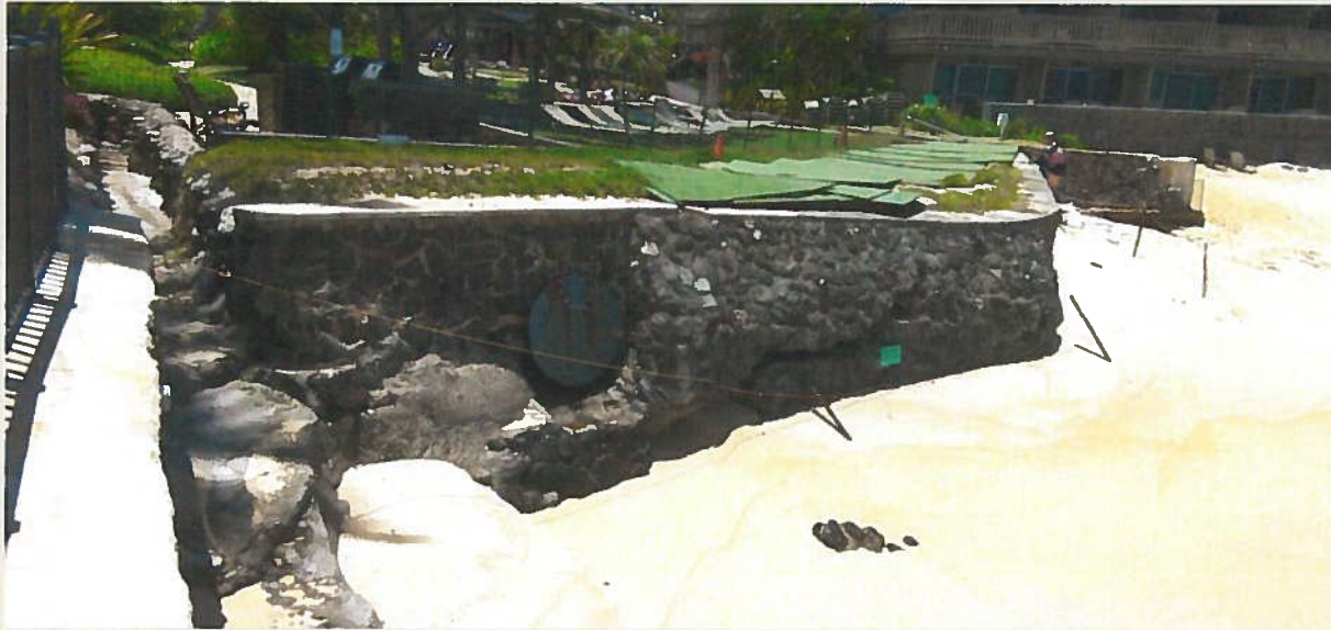
5. Looking at existing drainage outfall at seawall.
