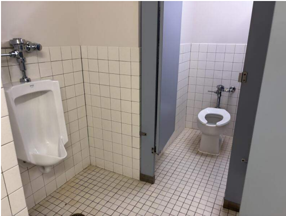
25 Typical men's restroom on each floor
