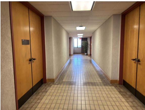
21 Typical common use corridor
