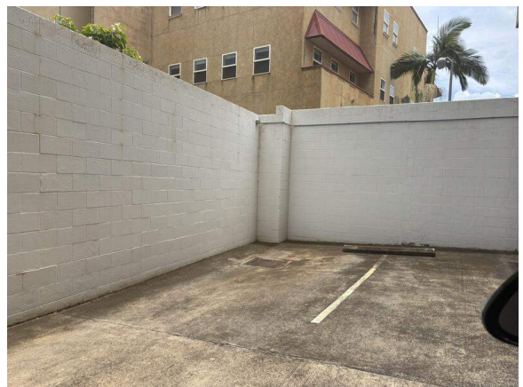
12 Site drain at parking area
