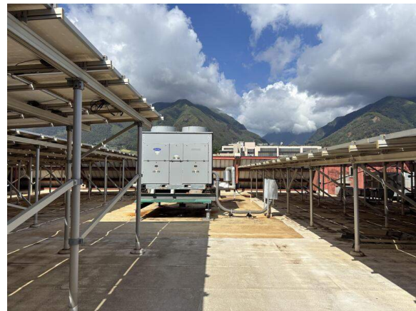
16 Overview of roof
