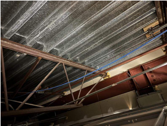
19 Underside of typical upper level
