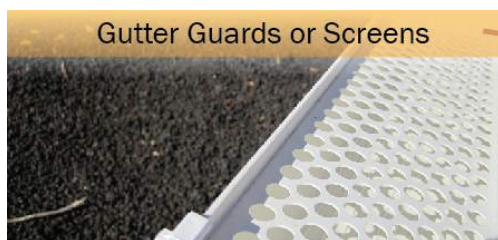
Figure 37. Rain gutters should have screens to keep leaf debris from accumulating. Maintain gutters to keep them clear and clean.
