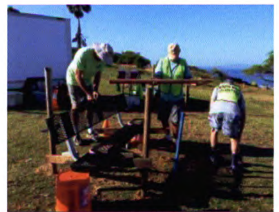
Phase II Bench Installation, Kamaole Beach Park
