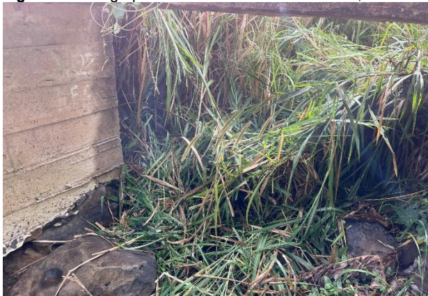
A) Upstream view of East Kuiaha Stream above Kauhikoa Ditch.
