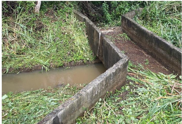
D) East Kuiaha Stream bypass over Kauhikoa Ditch.
