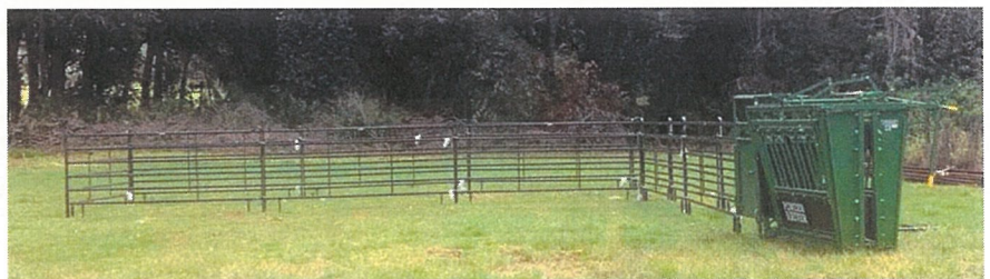
Figure 8. Preliminary site work completed for installation of corral / covered
