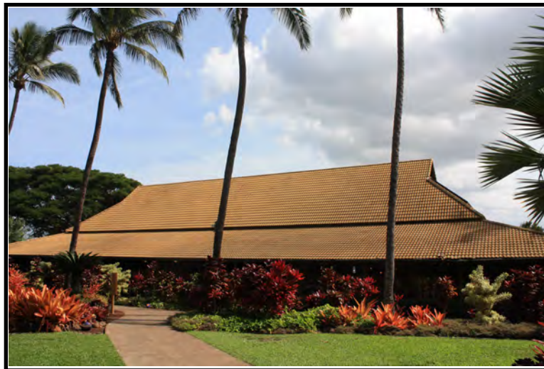
12. Looking east (makai) at the rear of the Maui Tropical Plantation Visitor Store from the village green.
