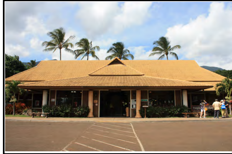
8. Looking west at the entrance to the existing Maui Tropical Plantation Visitor Store.
