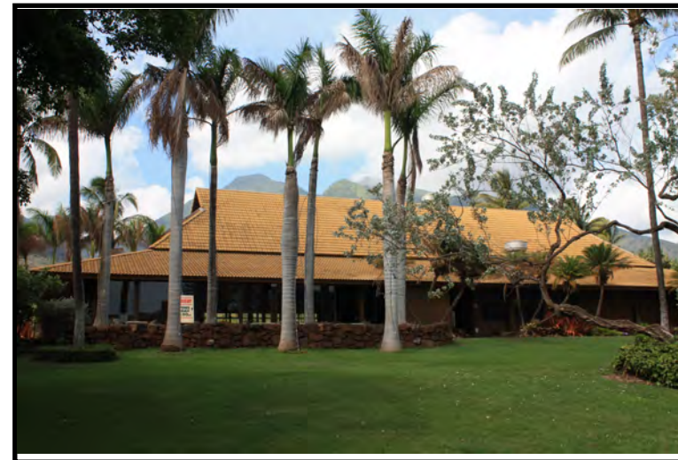
14. Looking west (mauka) at the restaurant / special events hall from the village green.
