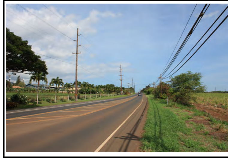
2. Looking north along Honoapi'ilani Highway towards Waikapū Town fronting the project.
