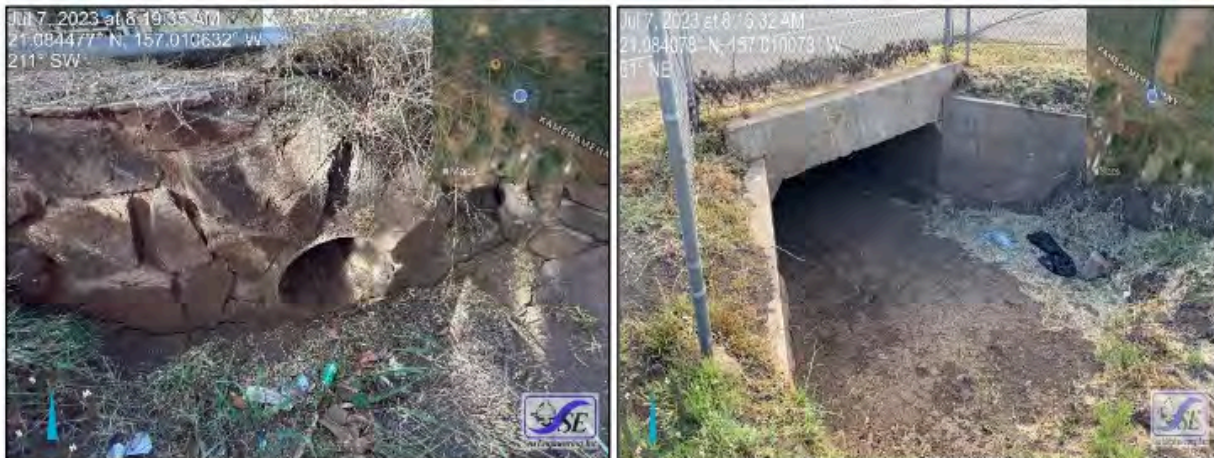
Figure 3-150. Drainage pipes to carry flow under Kamehameha V Highway mauka to makai.
