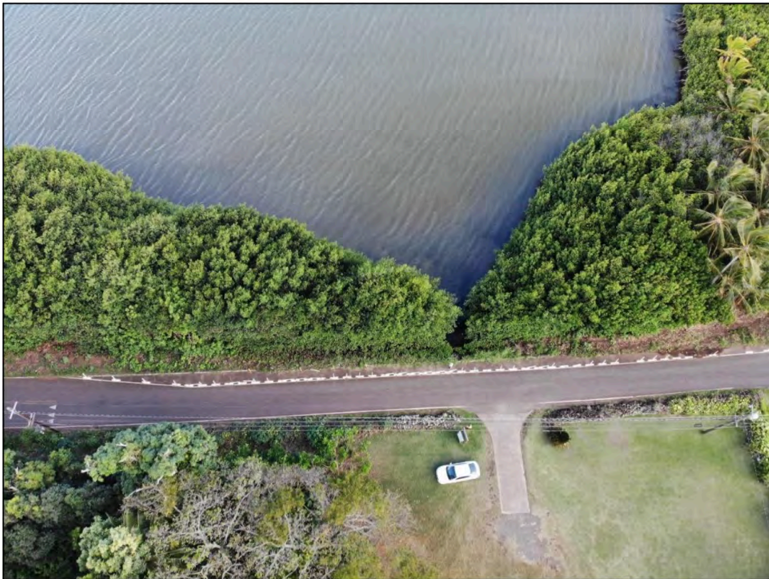
Figure 3-141 Our Lady of Seven Sorrows water at the one-lane road edge with a 5.75-foot erosion scarp down to the water surface
