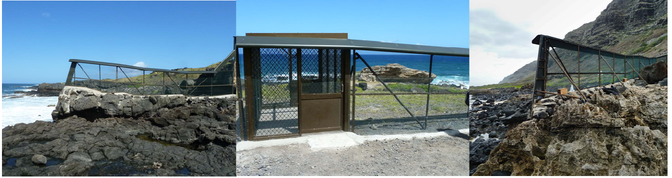
Figure 1.4: The south coastal end (left), center gate and north coastal end (right) of the fence.
