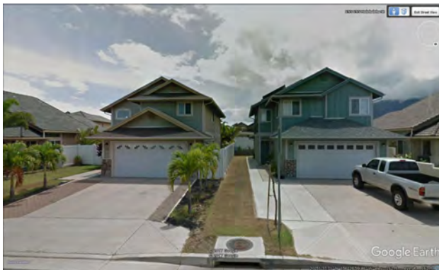
No more than 20% of single-family residences upon each side of a block's frontage may have front loaded garages.
