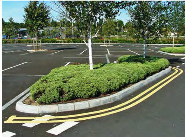
Canopy street trees in parking lots create shade and mitigate the heat island effect..
