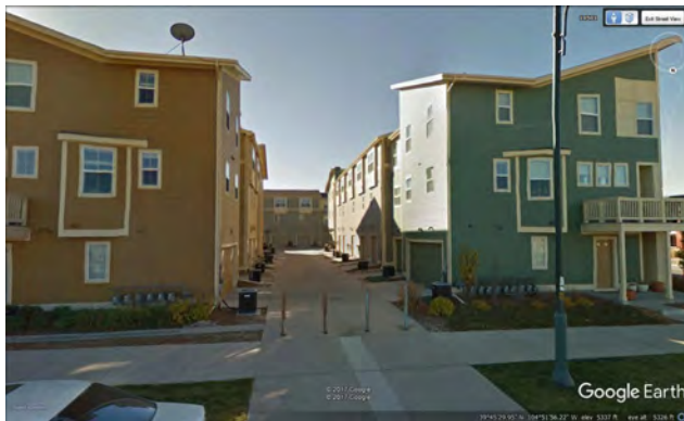
Alleyway serving townhomes. Stapleton, CO.
