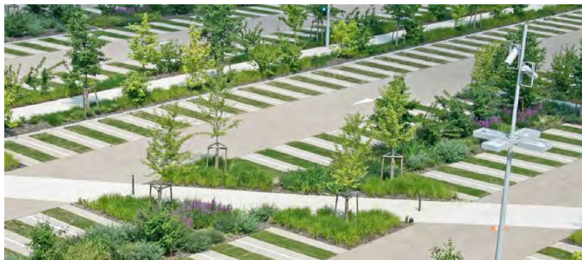
Alternative parking lot designs that minimize impervious surfaces through the use of grass parking systems are encouraged provided that they are sufficiently durable for the proposed usage and are adequately maintained.
