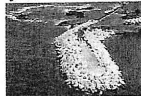
Kaumalapau harbor and breakwater the service. Even with a highly-trained professional staff and a much improved breakwater, there will be, in rare circumstances, conditions under which bringing in or keeping a 3,500-ton barge at the pier in this particular harbor will be too dangerous. As an indication that we must always respect the power of the ocean, on June 5, 2013, with the barge at the pier, three mooring lines, with a diameter of 1 3/4 inches and a breaking strength of 275,000 pounds, were parted (snapped) as a result of wave energy generated by large south swells. As Lanai residents are aware, the captain of the YB tug determined that conditions were too unsafe for the barge to remain in the harbor. We regret and apologize for the difficulty this necessary decision caused for Lanai residents, as well as the many visitors to the island that week. We hope this article helps all concerned to understand that decision.
