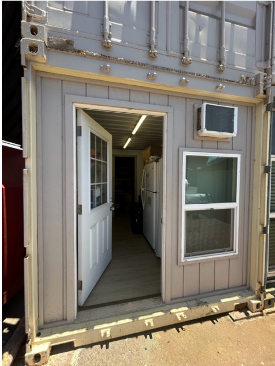
Figure 7. Shows exterior of food prep kitchen build in a shipping container.
