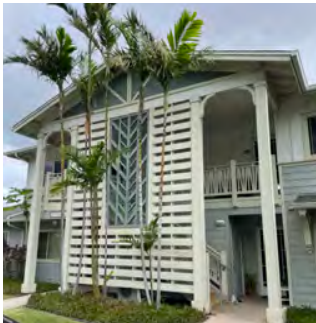
Figure 2.7 Example of projecting porch MMH frontage in Maui. Two-story units in the building are accessed by a single, shared entry that leads to a hall or small lobby area.
