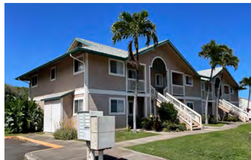
Figure 2.3 Density comparisons for different MMH types. A similar building size can vary in terms of density, because of additional units being provided within the same building envelope.
