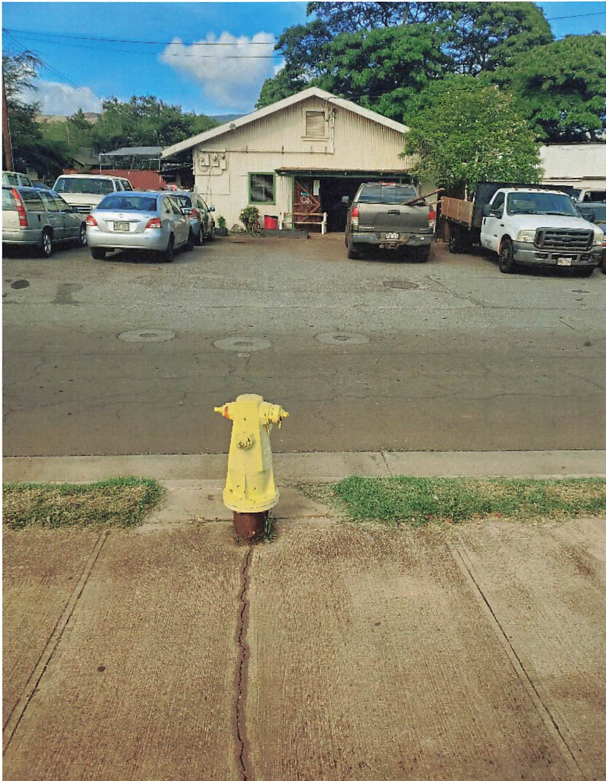
Fire Hydrant "B" looking to the front door of The Olde Laundrymat, which equals a distance of approximately 74'
