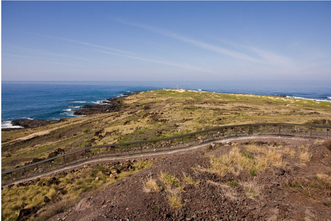
Figure 1.3 – Installed fence section at Ka`ena Point
