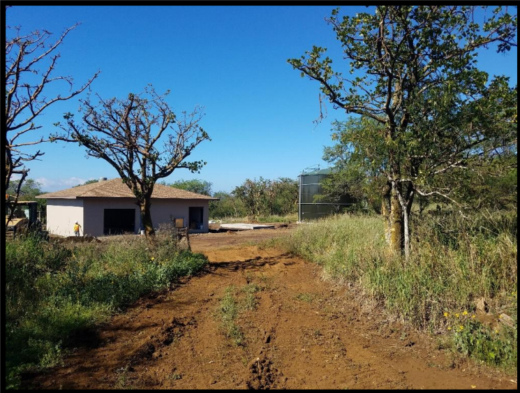
(2) 2-1-005:024 (State of Hawai'i) – Accessed and graded State land without permits to transport rock crushers to the site.
