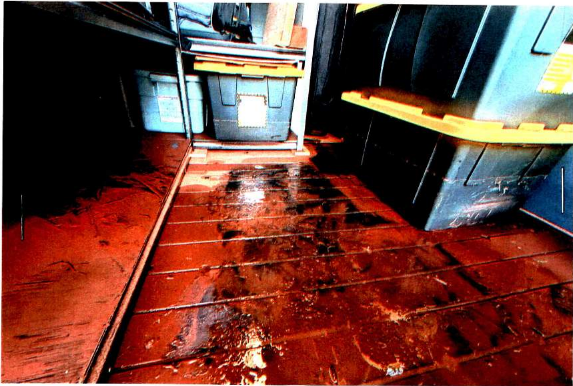
Damaged & warped press wood shelves
