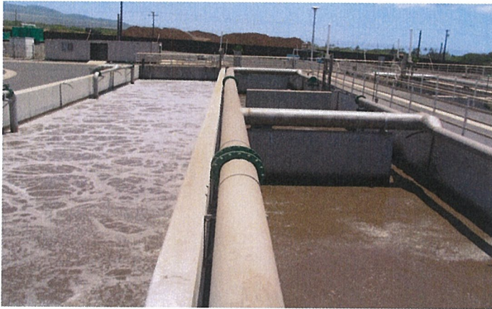
Figure 3: Kihei WWRFF Flexible Aeration Basin
