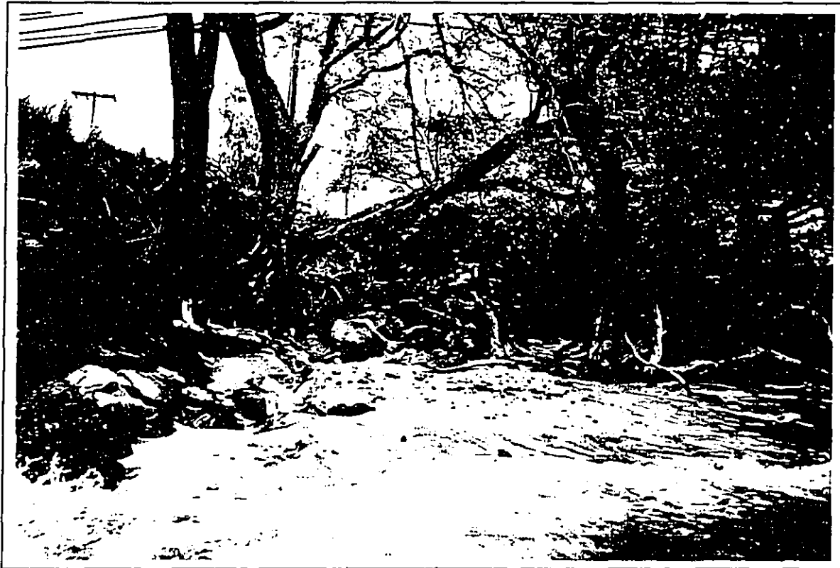
Figure 24. Location of Drain Outlet No. 3.
