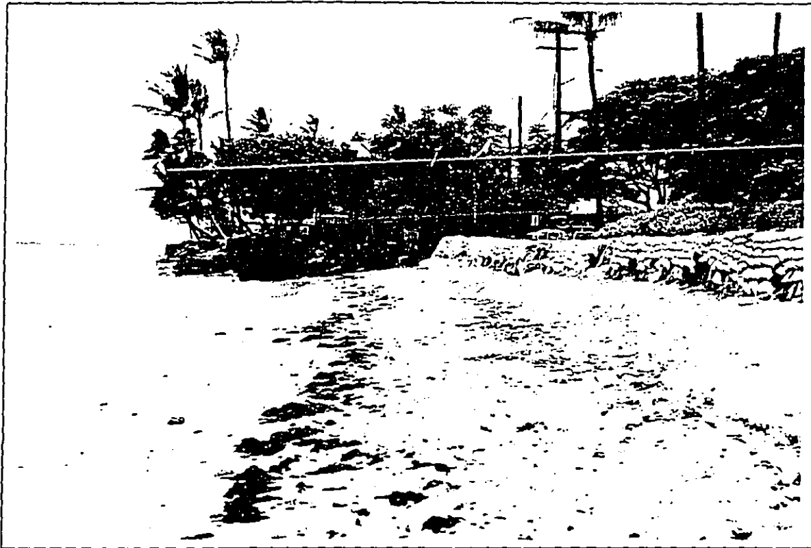
Figure 6. View of Drain Outlet No. 1 location, looking north on Kahana Beach.
