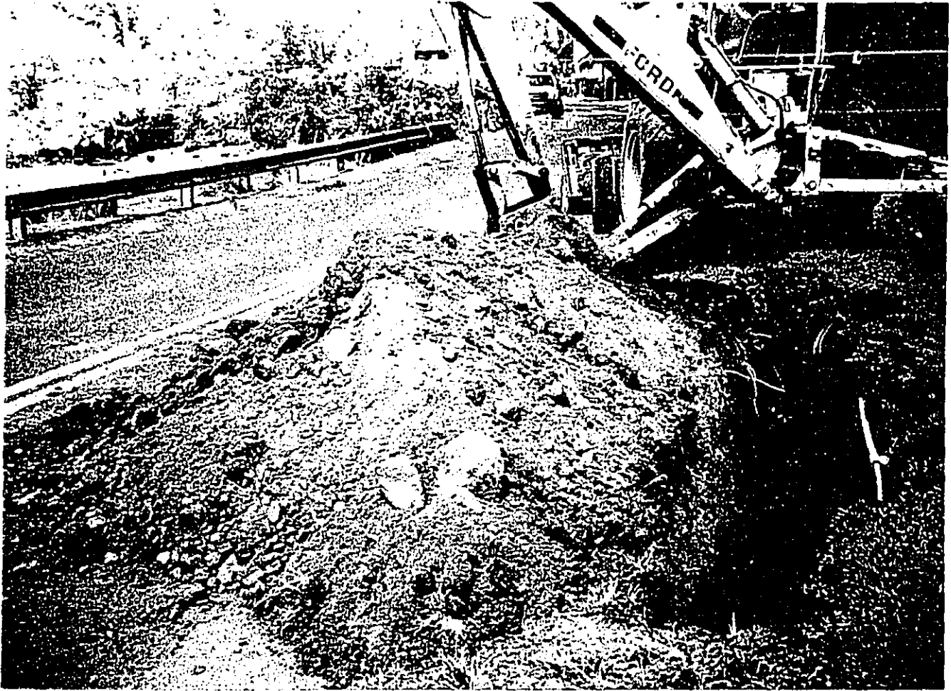
Photo 5 – BT 4—again illustrating the difficult working conditions.
