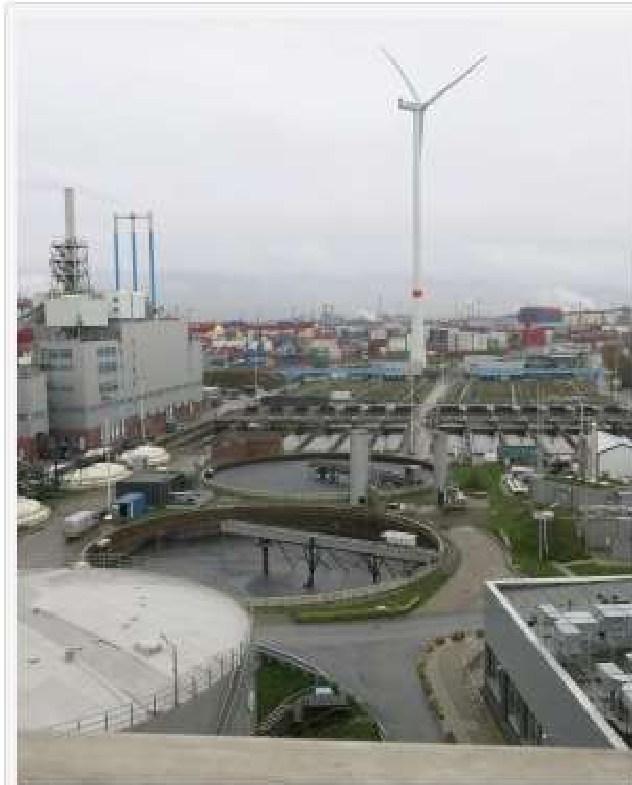
One of the plant's three windmills in the background, with the incinerator on the left.
