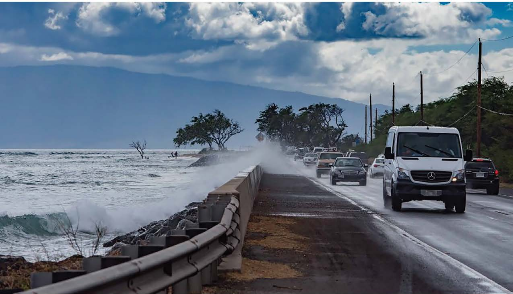
King Tide Flooding Honoapi'ilani Highway (2017)
