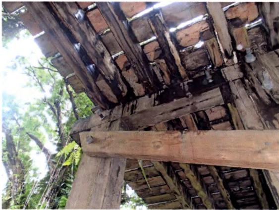
PHOTO 4 6x12 TIMBER GIRDERS LAPPED OVER INTERMEDIATE PIER
