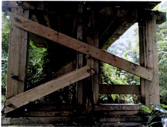
PHOTO 5 TIMBER PIER BETWEEN THE MAUKA AND MAKAI SPANS
