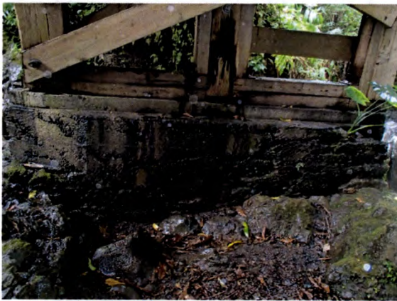
PHOTO 6 CONCRETE PIER WALL
