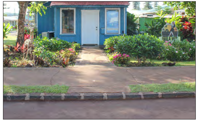
The roads surrounding Dole Park are more elaborate than those leading to the historic residential areas. They are wider and they have basalt stone curbs and concrete sidewalks.
