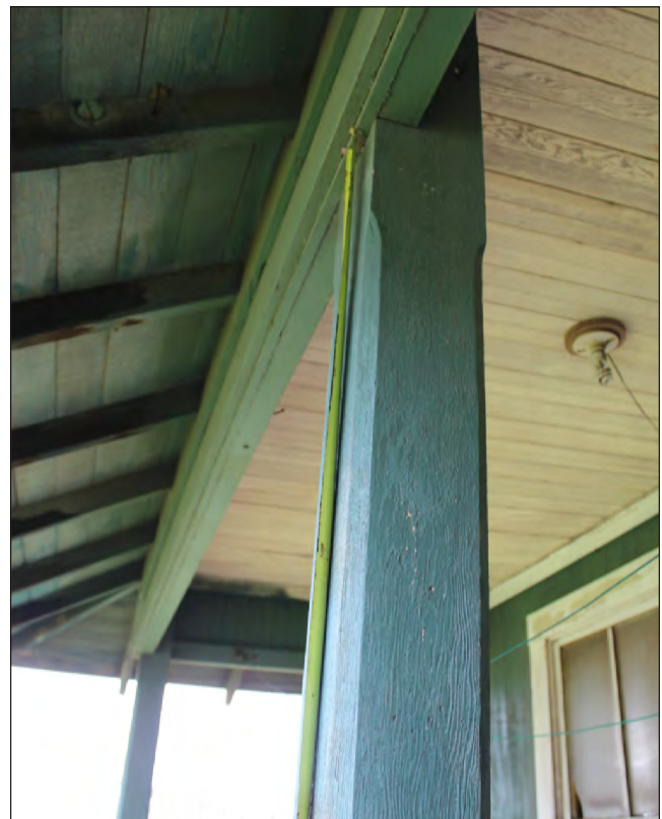
Exposed Rafter Tails, Porch Columns, and Ceiling
