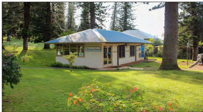
Many commercial buildings are fronted by lawns or landscaped areas.
