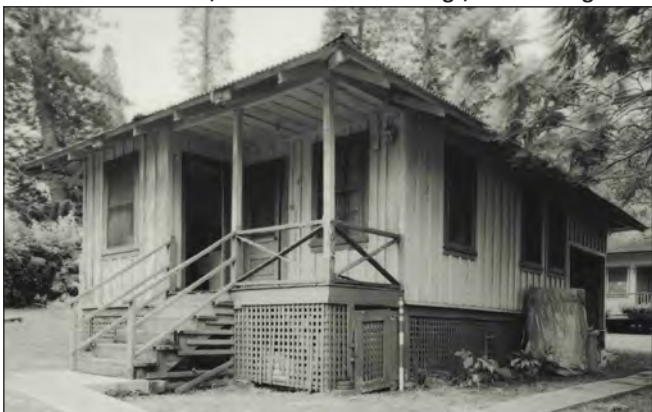
Porch Columns, Balustrades and Railings, and Skirting
