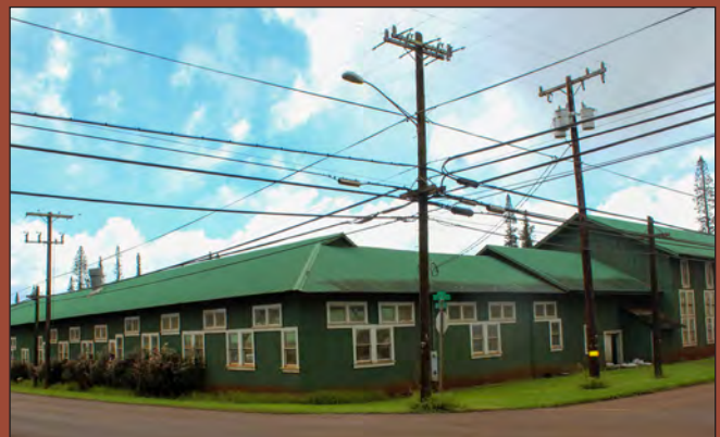
Overhead utility lines are allowed in the Country Town Business District.
