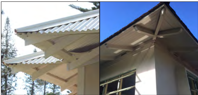
Exposed Rafter Tails
