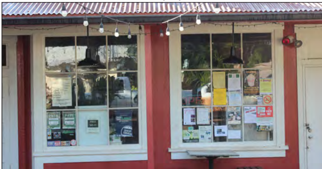
Storefront Display Windows
