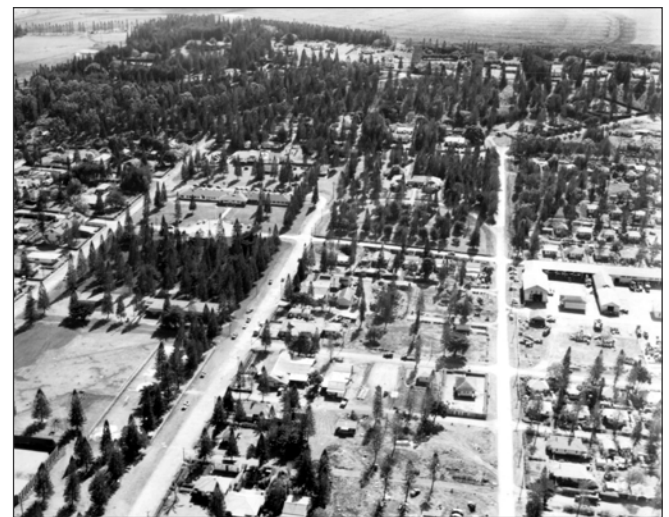
Ca. 1950 aerial photo of Lāna'ī City, looking toward the former Dole Administration Building. Photo: Lāna'ī Culture & Heritage Center.
