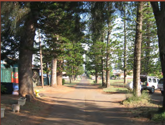
Road widening is not required. Work on existing buildings and new construction are exempt from the road widening requirements in the Maui County Code. Photos: Stanley Solamillo.
