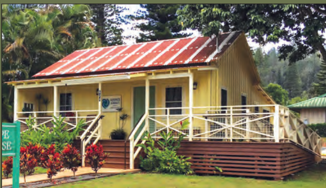
This access ramp is simple in design and its foundation and railings match the historic building. Photo: Generations Magazine.
