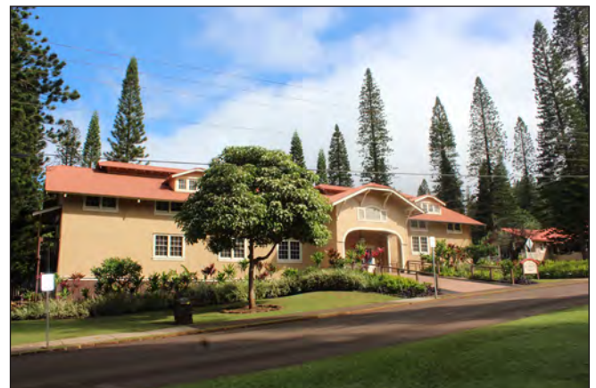
Many roads drain due to the town's naturally sloping topography.
