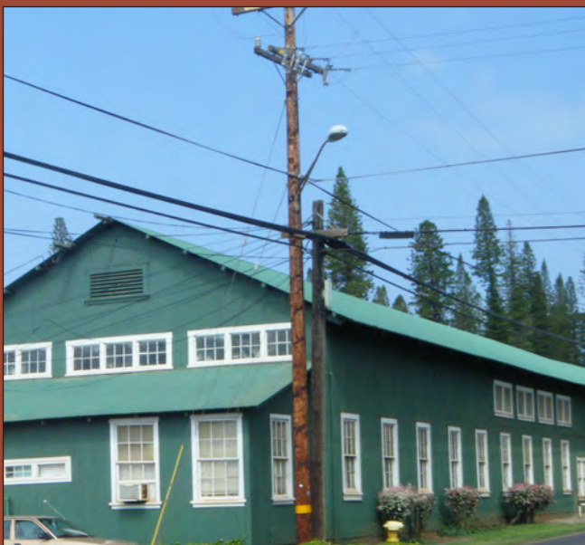
All of the historic street lights in Lāna‘i City have been replaced with these modern “cobra head” fixtures. As these fixtures reach the end of their lives, consideration should be given to installing new fixtures that are more historically accurate and compatible with the character of the town. Photo: Stanley Solamillo.
