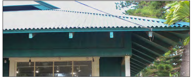
Deep eaves and exposed rafter tails are common roof features in Lāna'ī City.
