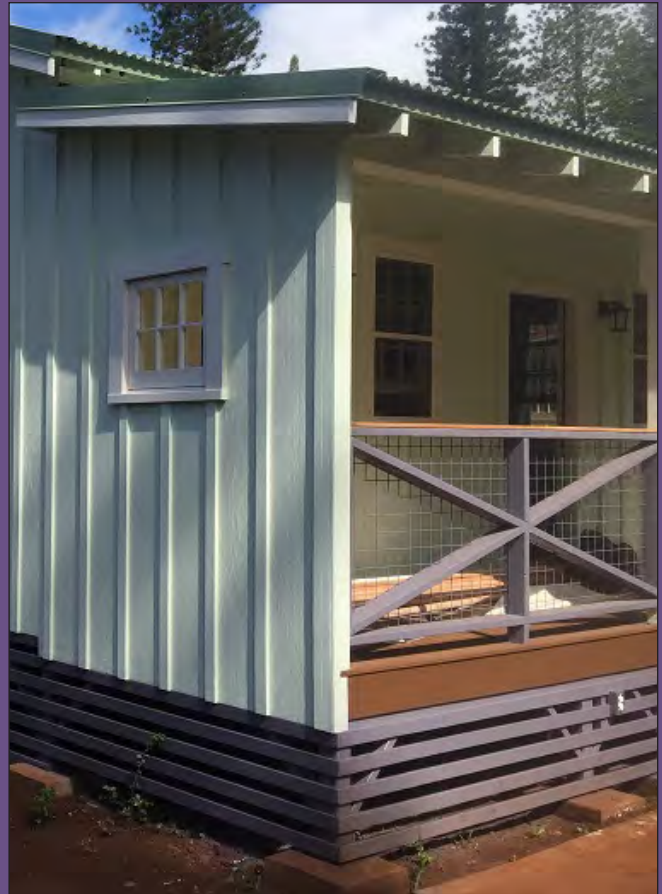
This new home's front porch is similar to the porches of neighboring historic buildings in terms of massing, proportions, materials, and details. Photos: Glenn Mason, Mason.
