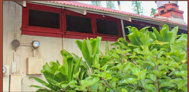
Maintain a buffer between the building and landscaping to prevent moisture damage.
