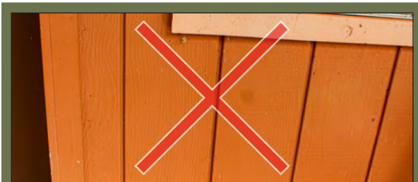
Do not cover original siding with T 1-11.
