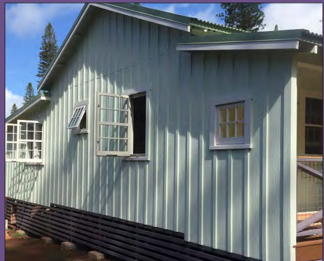
The this new home's board and batten siding resembles the appearance of siding traditionally found in Lāna'i City. Photo: Glenn Mason, Mason.
