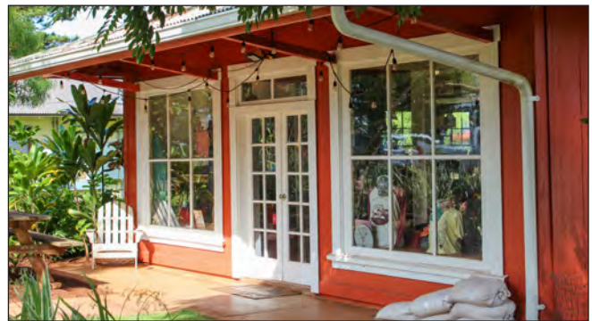
Many commercial buildings have front porches and lack parapets.
