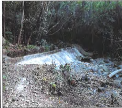
Figure 28: S. Waikapū Dam Intake Diversion (2012)
