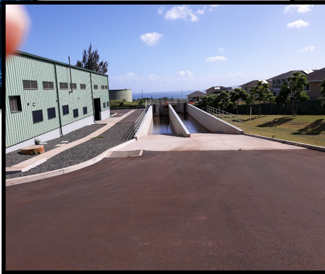
6 Surface Water Treatment Facilities
