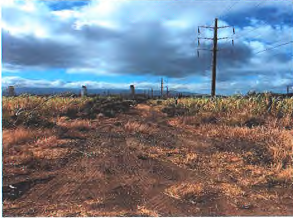
Transmission Corridor Next to Pohakea
