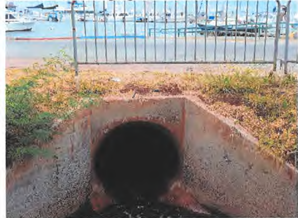
Culverts Discharging into Harbor
