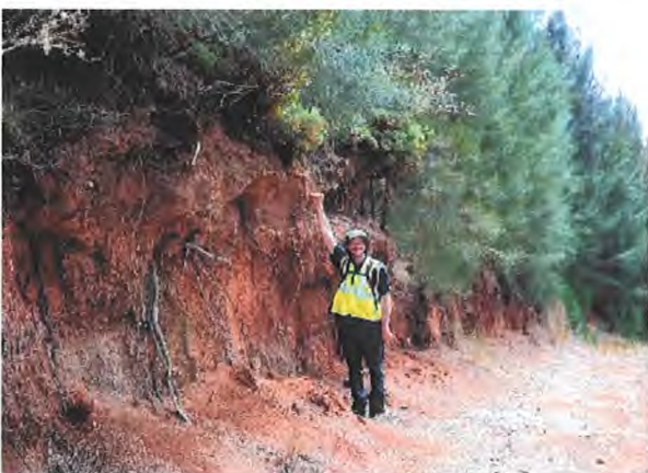
Exposed Soil Along Road
