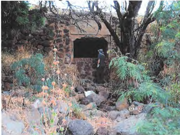
Culverts Discharging into Harbor
