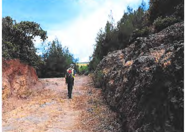
Exposed Soil Along Road
