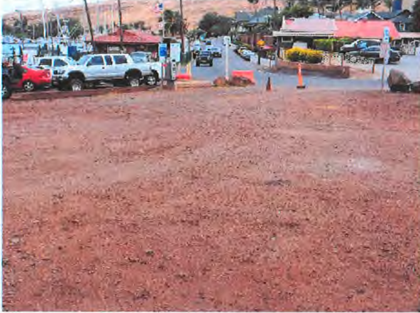
Dirt Lots with No BMPs in Place
