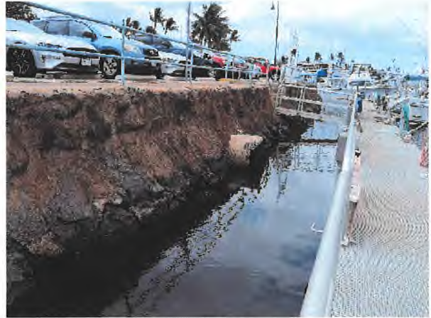
Culverts Discharging into Harbor
