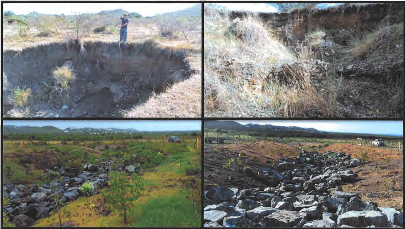
Figure 22. Examples of Head Cutting and Stabilization
