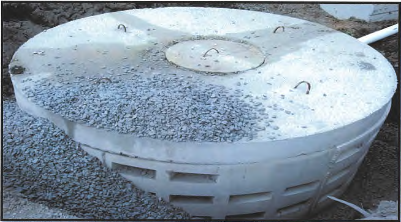
Figure 28. Stormwater Infiltration Well
