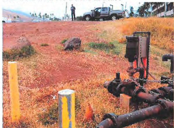
Dirt Lots with No BMPs in Place
