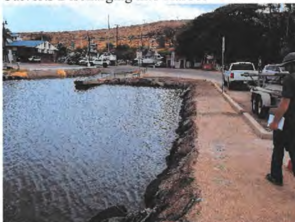
Culvert Outfall to Harbor
