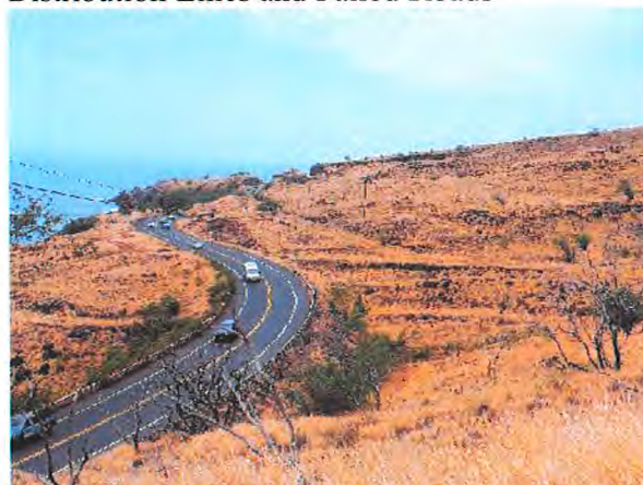
Transmission Lines along the Pali
