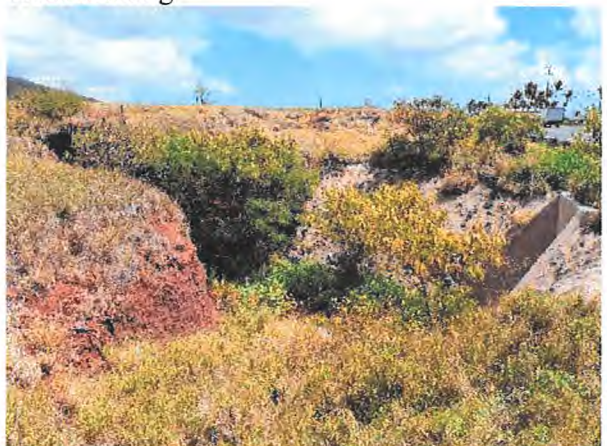
Culvert Backwall and Head Cutting
