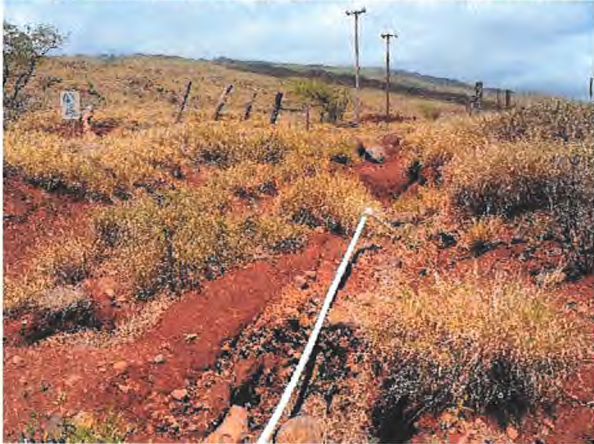
Channelization and Erosion
