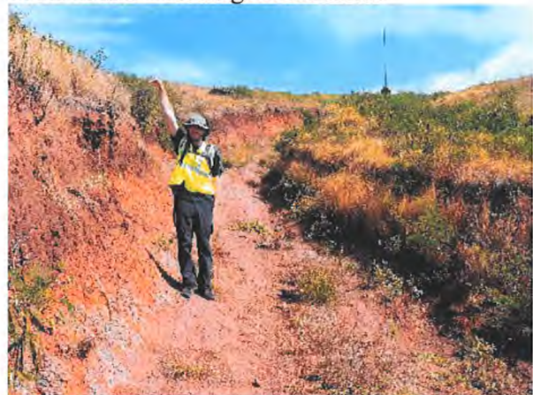
Exposed Soil Along Road
