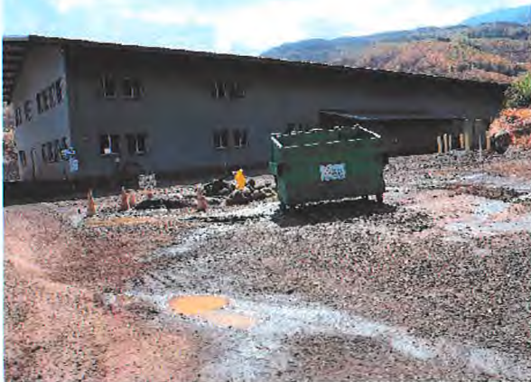
Gravel Roads with Mud and Erosion
