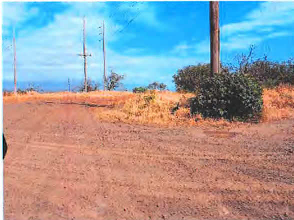
Gravel Roads Near Ditches
