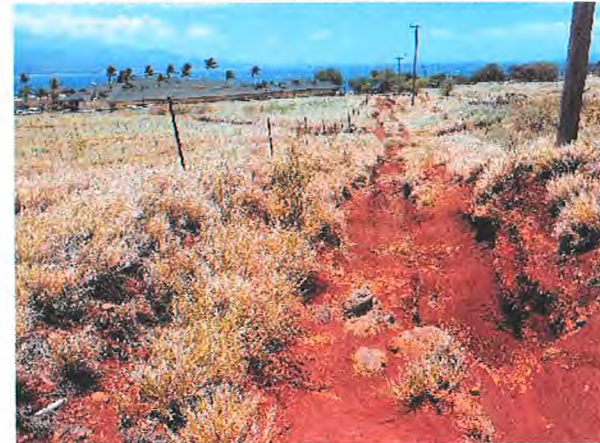
Distribution Lines and Failed Roads
