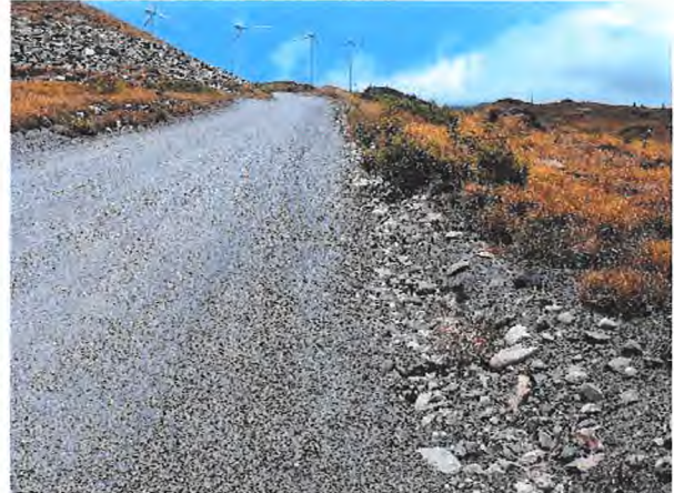
Well Maintained Road with Swale
