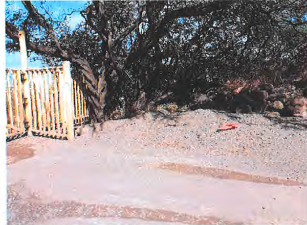
Gravel Piles Near Entrance
