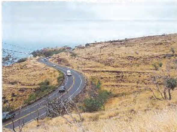
Transmission Lines along the Pali
