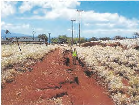
Distribution Lines and Failed Roads
