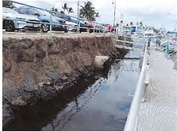
Culverts Discharging into Harbor
