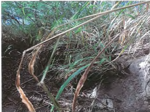
Exposed Stream Banks within Pohakea
