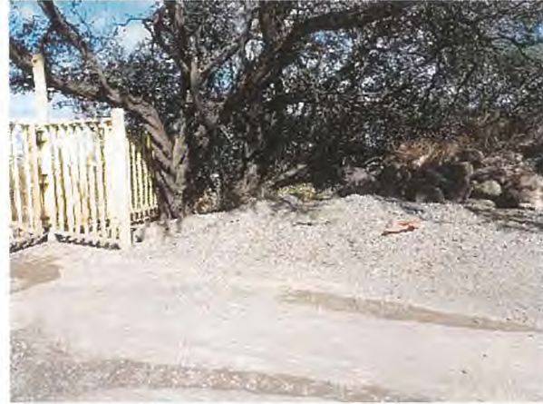
Gravel Piles Near Entrance
