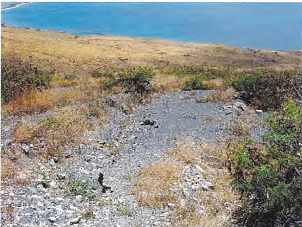
Gravel Loss at Kickouts
