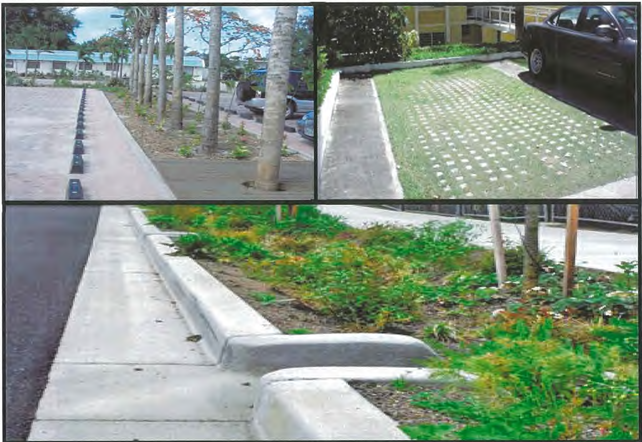
Figure 31. Examples of Low Impact Design (LID) Stormwater Treatment in Parking Lots
