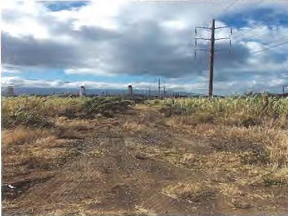
Transmission Corridor Next to Pohakea
