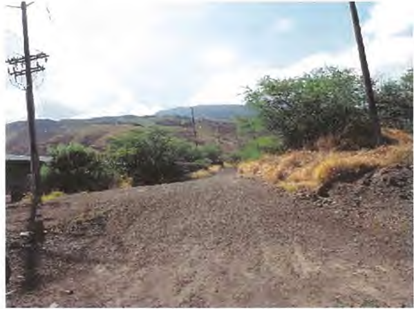
Gravel Roads Near Ditches
