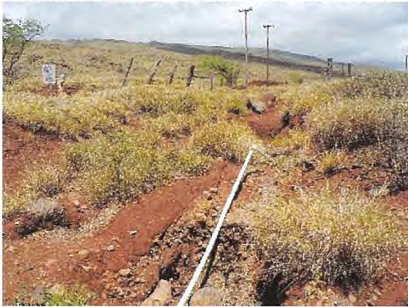
Channelization and Erosion
