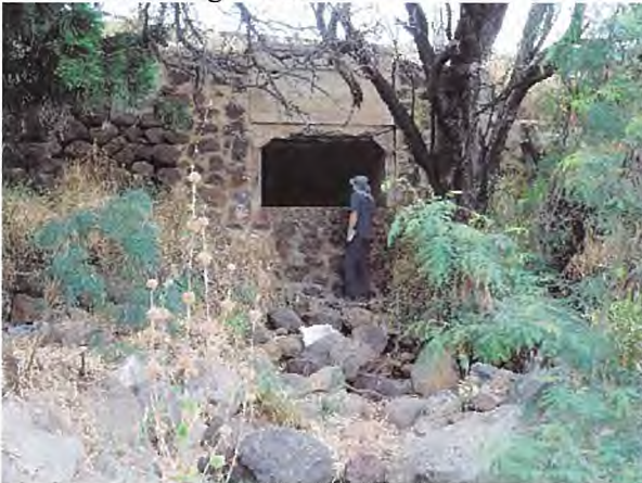
Culverts Discharging into Harbor
