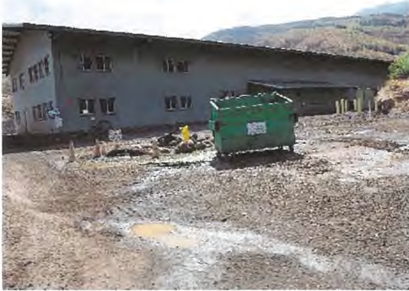
Gravel Roads with Mud and Erosion
