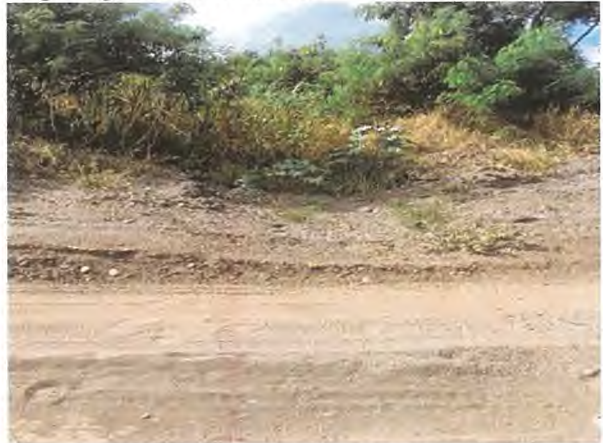
Road Crossing Pohakea Lacking BMPs
