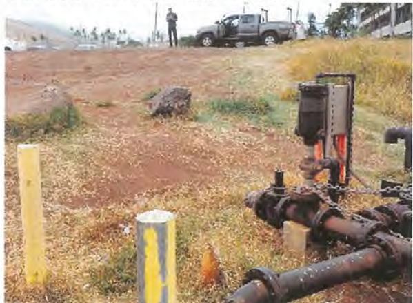
Dirt Lots with No BMPs in Place
