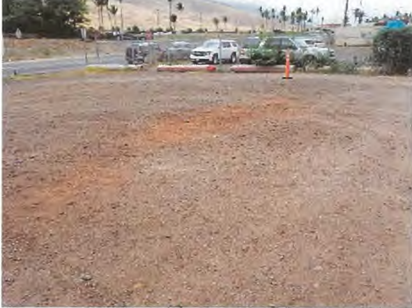
Dirt Lots with No BMPs in Place
