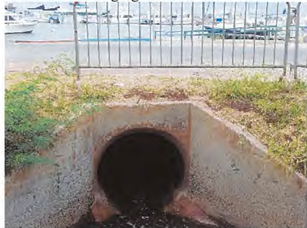
Culverts Discharging into Harbor
