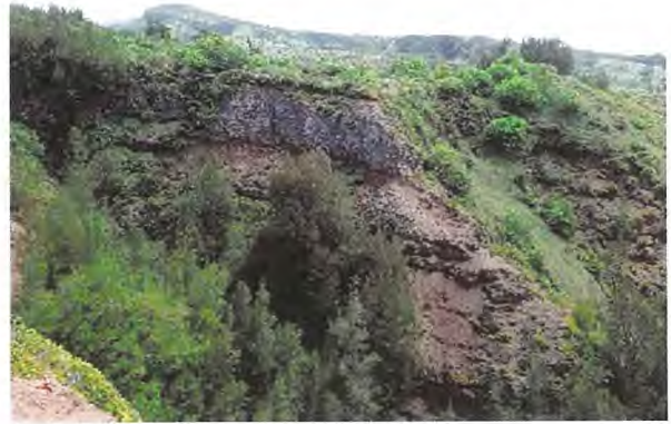
Loss of Vegetation
