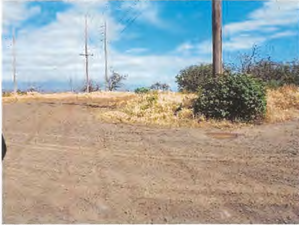
Gravel Roads Near Ditches
