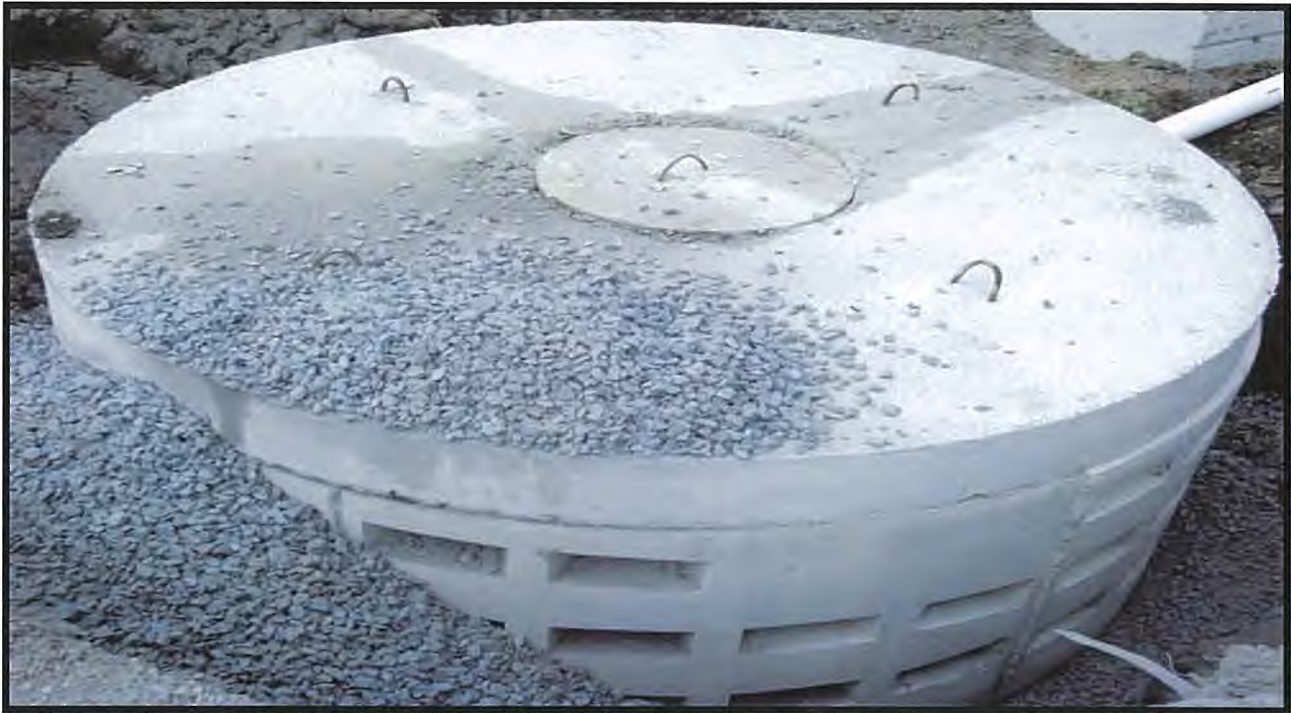
Figure 28. Stormwater Infiltration Well
