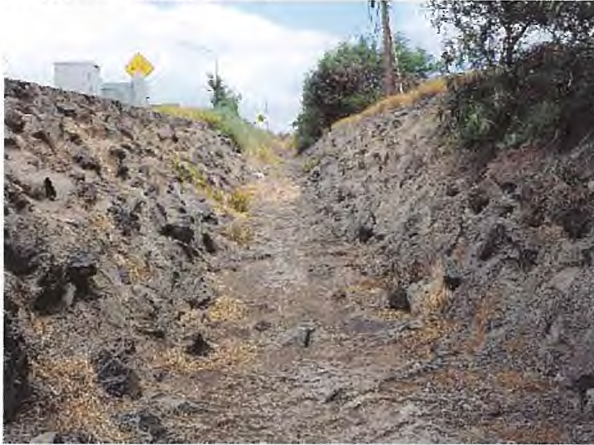
Waihe'e Makai Ditch – Armored and Box Cut
