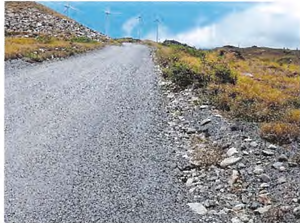
Well Maintained Road with Swale
