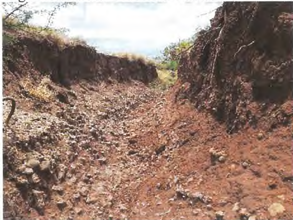
Highly Eroded Stream Channel
