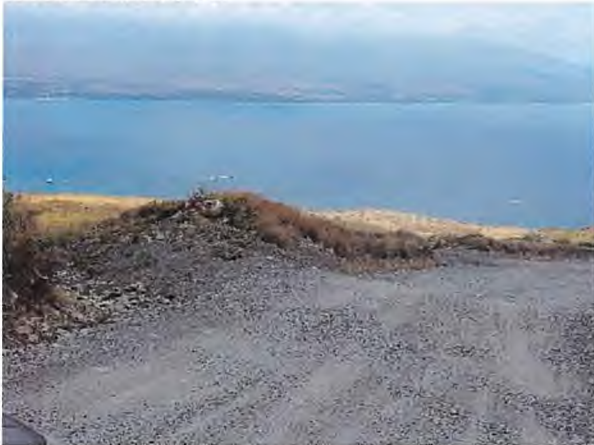
Water Bars and Kickouts
