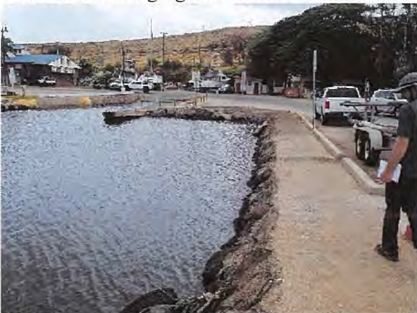
Culvert Outfall to Harbor
