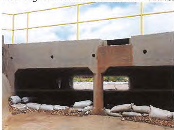
Sand Bags Under Hau'oli Street
