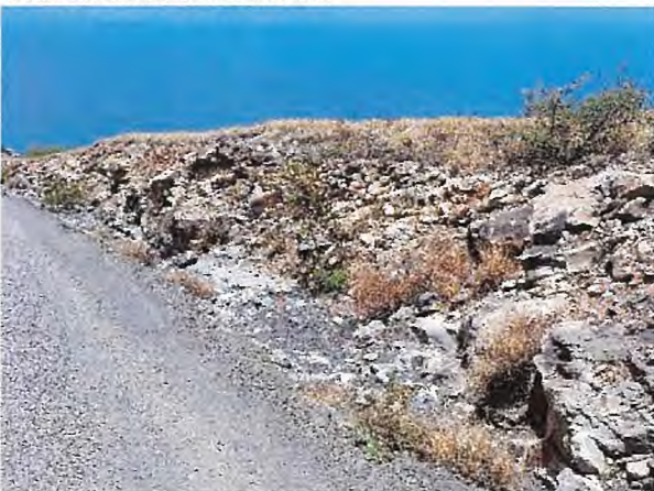
Channelization and Gravel Loss in Swale
