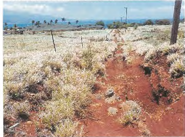
Distribution Lines and Failed Roads
