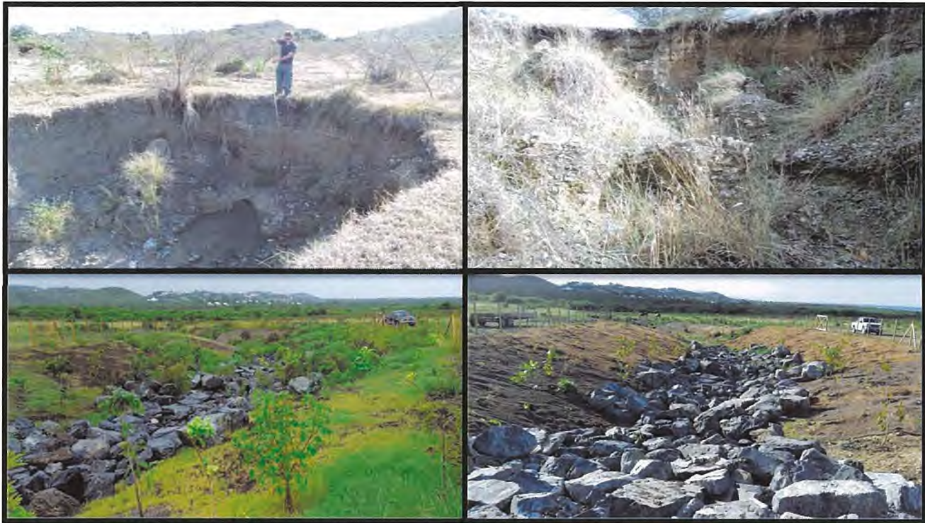
Figure 22. Examples of Head Cutting and Stabilization
