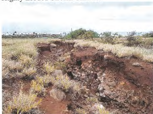
Highly Eroded Stream Channel
