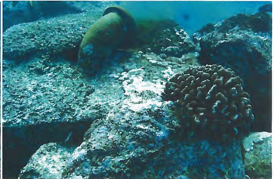
EXHIBIT 1. Photographs of ocean discharge diffusers in Hilo Bay off the Hilo Wastewater Treatment Plant (top) and off Sandy Beach off the East Honolulu Wastewater Treatment Plant (bottom). Both diffusers are at a water depth of approximately 35-40 feet. Concentrated streams of treated effluent of high nutrient concentration, low salinity, and elevated temperature relative to receiving water can be clearly seen in both photos. Note presence of live corals on both outfall structures, lack of presence of filamentous algae, and clarity of water. Both ocean outfalls have been in operation since the 1970's. All photographs taken by S. Dollar.
