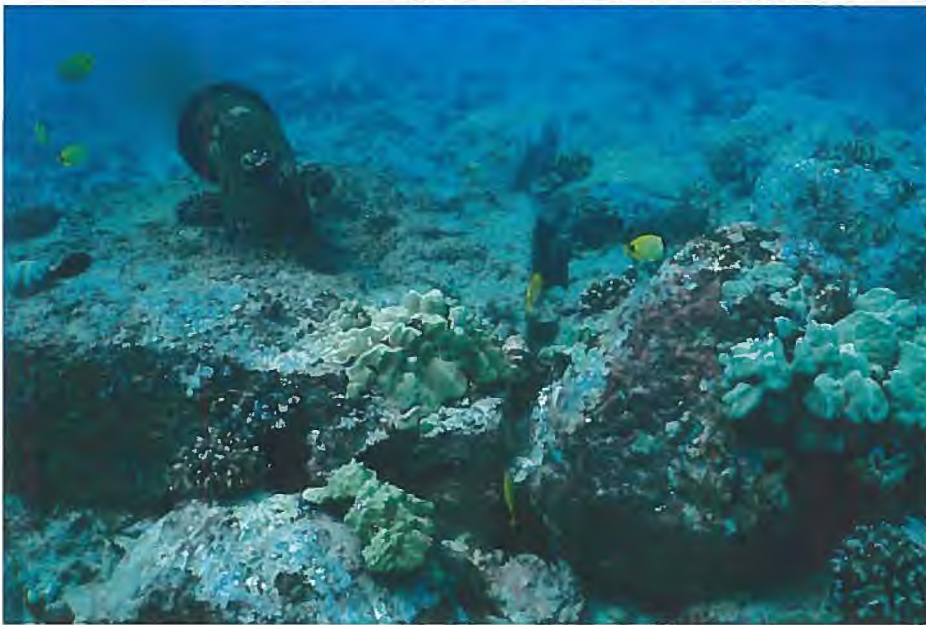
EXHIBIT 1. Photographs of ocean discharge diffusers in Hilo Bay off the Hilo Wastewater Treatment Plant (top) and off Sandy Beach off the East Honolulu Wastewater Treatment Plant (bottom). Both diffusers are at a water depth of approximately 35-40 feet. Concentrated streams of treated effluent of high nutrient concentration, low salinity, and elevated temperature relative to receiving water can be clearly seen in both photos. Note presence of live corals on both outfall structures, lack of presence of filamentous algae, and clarity of water. Both ocean outfalls have been in operation since the 1970's. All photographs taken by S. Dollar.
