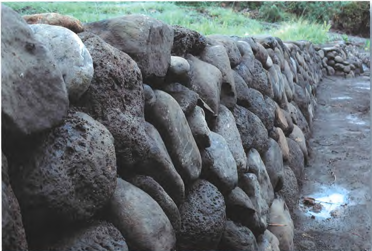
Figure 42: Lo‘i Kalo Wall Restoration at Noho‘ana Farm, Waikapū - Hōkūao Pellegrino (2005)
