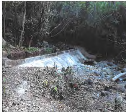
Figure 28: S. Waikapū Dam Intake Diversion (2012)
