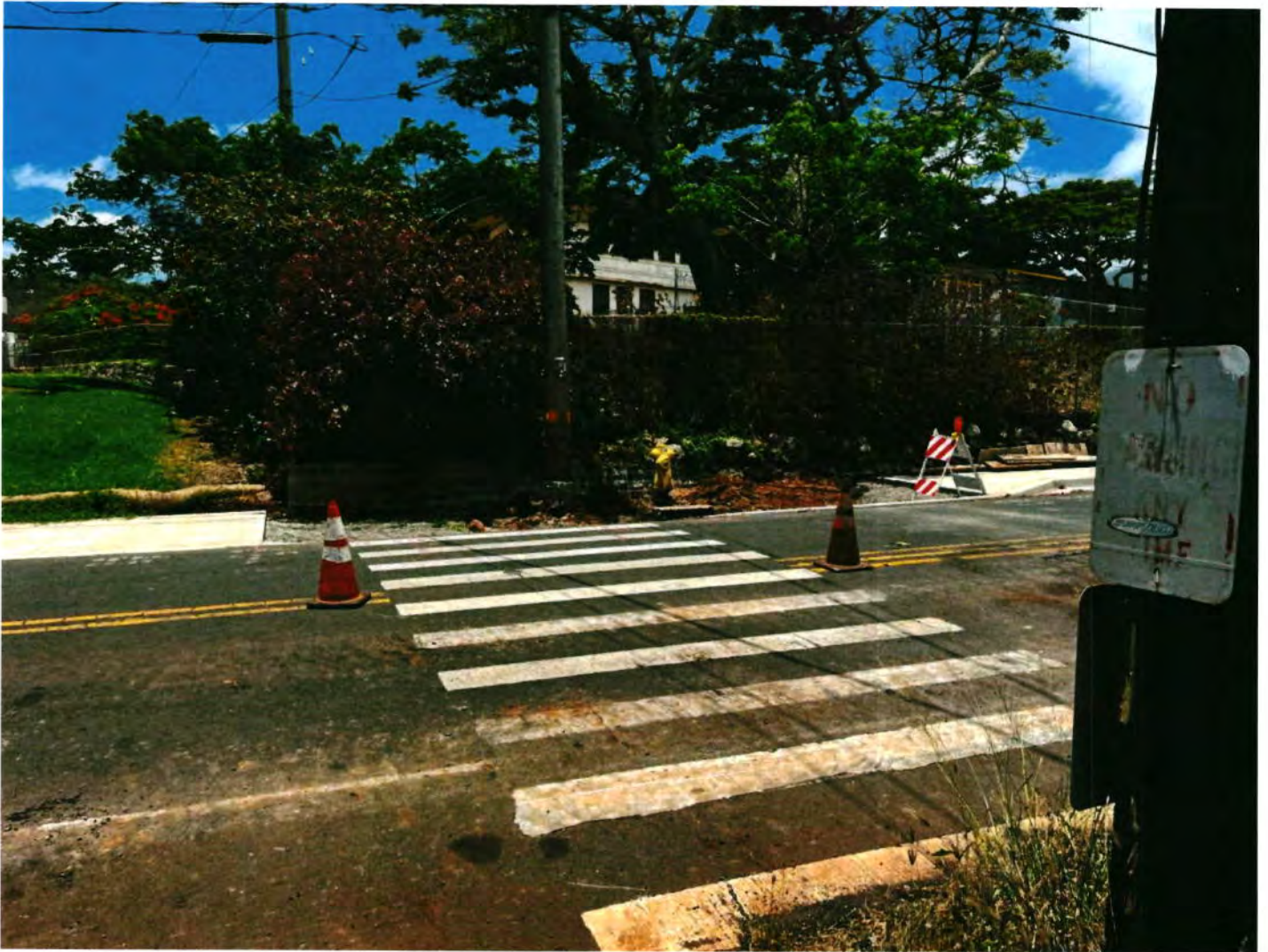
15 15-Insured's property Abutts Mill street
