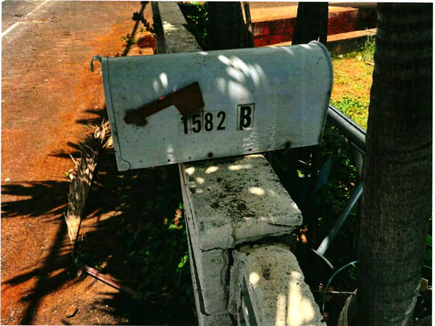
3 3-Loss Location Date Taken: 7/14/2022 Taken By: Kevin Frost
