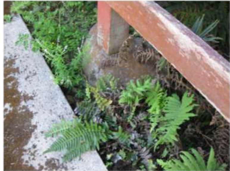
8. One of the Padstones Holding the Church Structure
