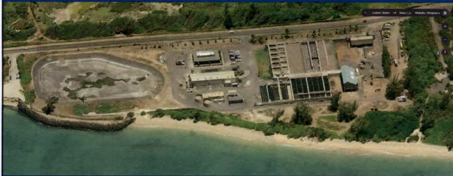
Wailuku-Kahului Wastewater Facility, circa 2011
