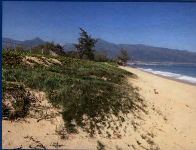
Wailuku-Kahului Wastewater Facility, 2016
