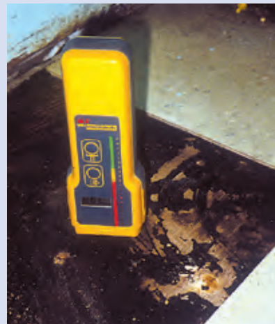
Photo 9: Moisture meter measuring moisture content of plywood subfloor
