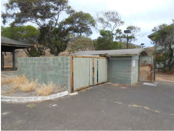
PTESB1: Overview of Trash Enclosure/Storage Building looking north.
