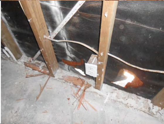
PB2D.2: Sole plate dry rot.
