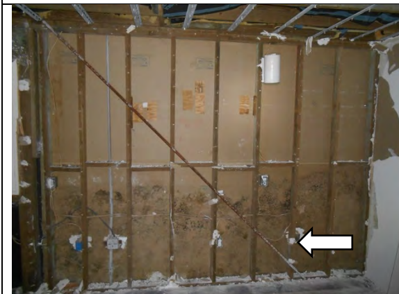
PA1CD.8: Discontinuous stud.
