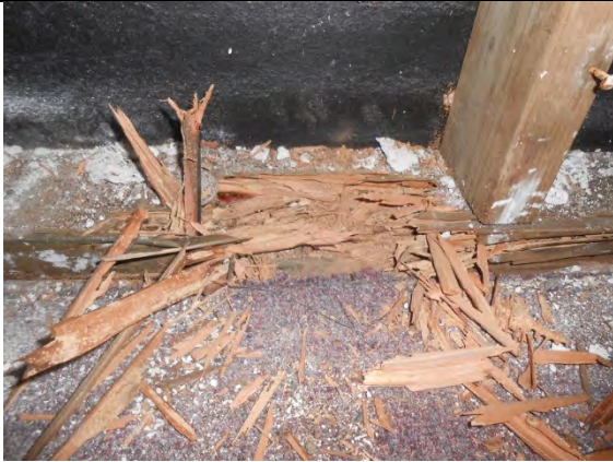
PB1D.1: Sole plate dry rot.
