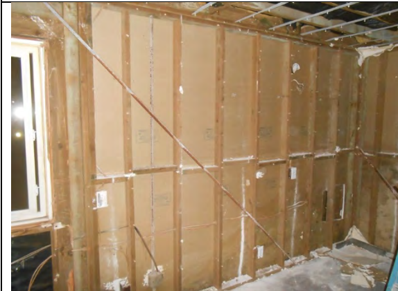
PB1D.6: Rusting steel wall braces.
