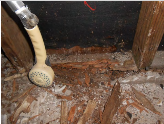
PA1D.4: Sole plate dry rot.
