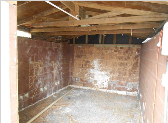
PTESB5: Interior view of storage building.
