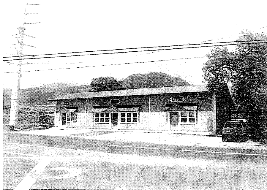
Building Fronting Waiale Drive.
