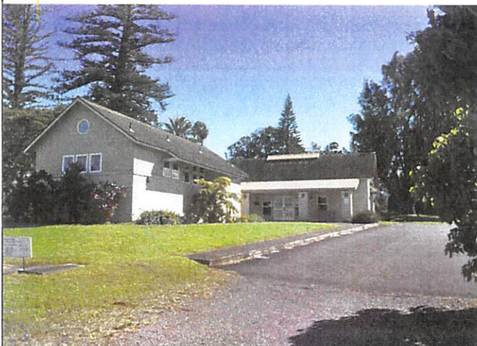
Restrooms and Children's Classroom (1999)
