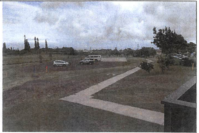
2016 gravel parking lot under construction
