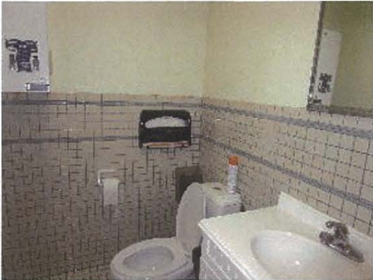
2nd Floor Interior
