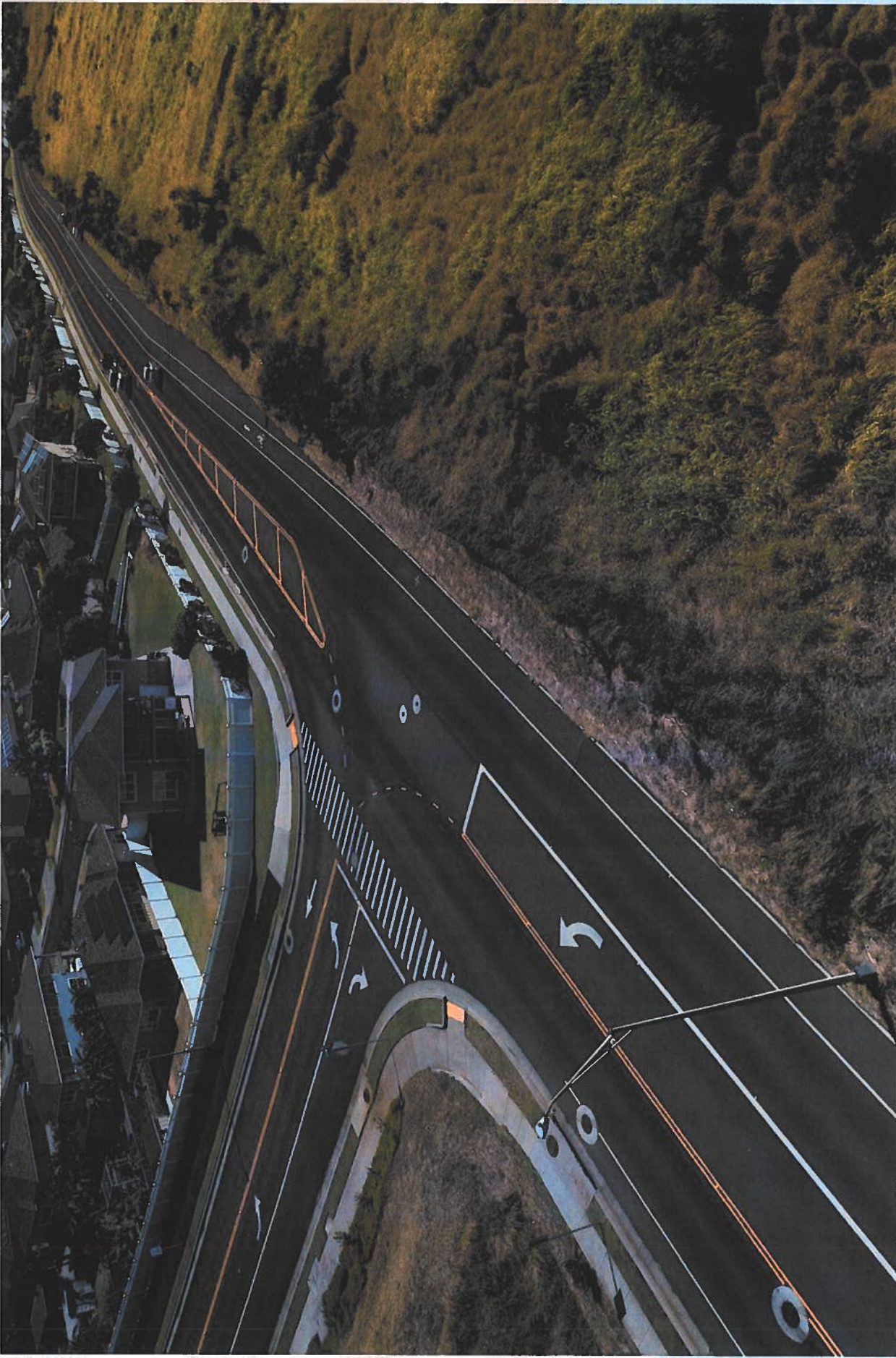
Existing Conditions at intersection of Ku'ikahi Drive and Kehalani Mauka Parkway
