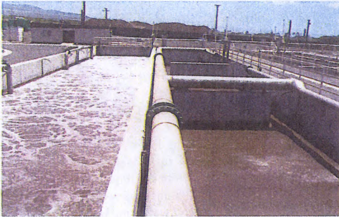
Figure 3: Kihei WWRF Flexible Aeration Basin
