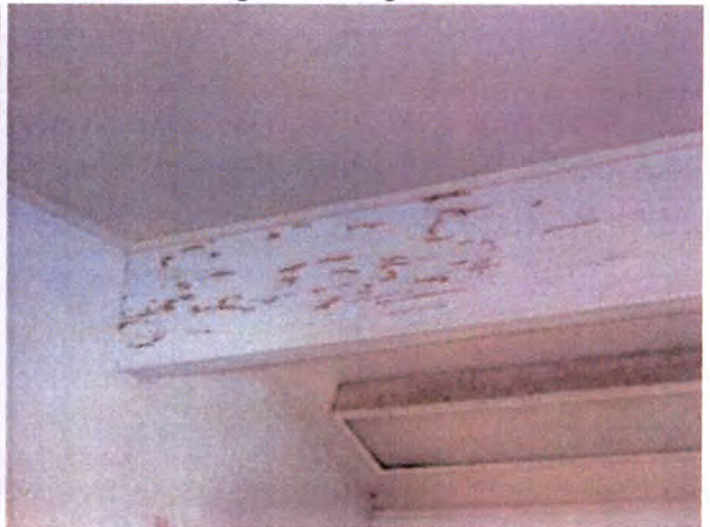
B-201: Ceiling joists were severely termite damaged and need to be repaired/replaced.
