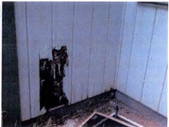
Visible indications of WDO (termite) damage noted. Recommend having a licensed pest contractor evaluate and treat as necessary. Also, recommend having a licensed contractor evaluate and repair/replace damaged material as necessary.
