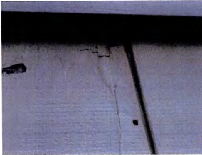
Visible indications of WDO (termite) damage noted. Recommend having a licensed pest contractor evaluate and treat as necessary. Also, recommend having a licensed contractor evaluate and repair/replace damaged material as necessary.
