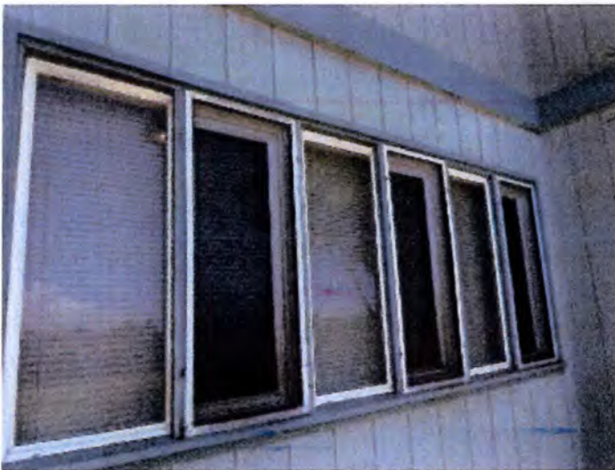
Vinyl framed windows noted
