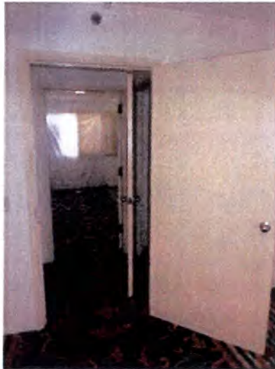
Bldg A doors operated when tested.
