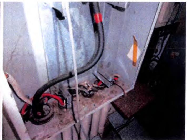
All of the branch wiring to buildings B and C was cut with circuit breakers removed. Recommend having a licensed electrical contractor repair.
