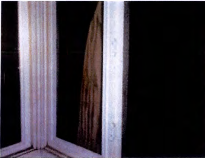
Many of the ground floor windows were broken at the time of inspection. Recommend replacement.
