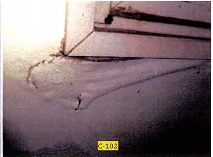
Most of the exterior facing lower interior wall finishes had moisture damage observed. Recommend removal and replacement of affected materials.
