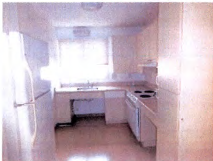
The kitchens in building A appeared to be functional at the time of inspection.
