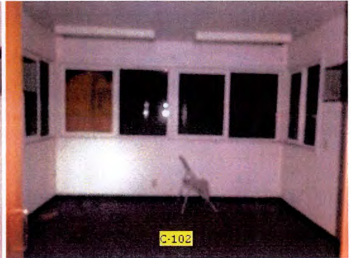
Each dwelling unit was serviced by two (2) sleeping rooms at the time of inspection.
