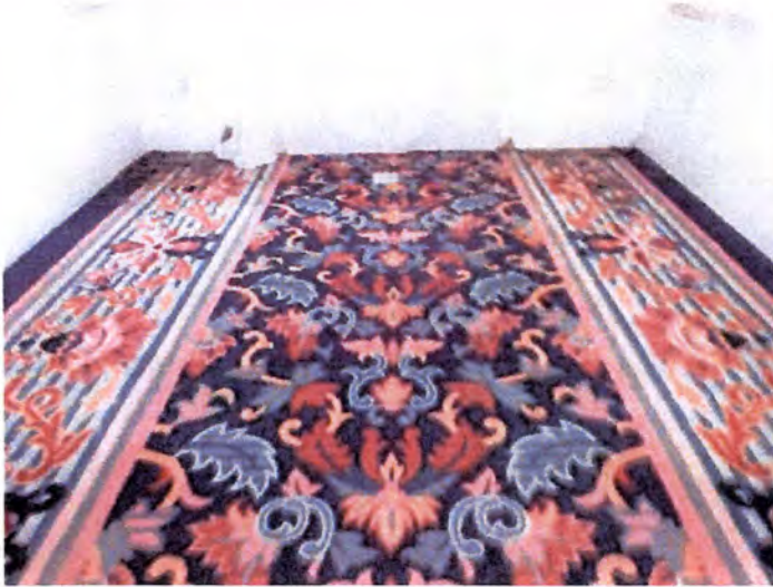
Bldg A Flooring appeared to be in functional condition at the time of inspection.
