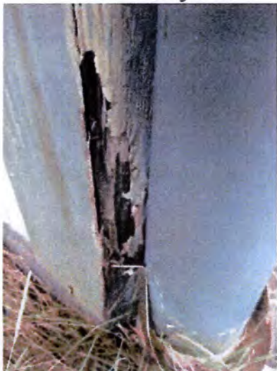
Visible indications of WDO (termite) damage noted. Recommend having a licensed pest contractor evaluate and treat as necessary. Also, recommend having a licensed contractor evaluate and repair/replace damaged material as necessary.
