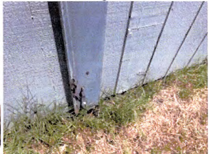
There were visible indications of WDO (Wood Destroying Organism) damage noted at the fascia and soffit areas. Recommend having a licensed contractor evaluate and repair/replace as necessary.
