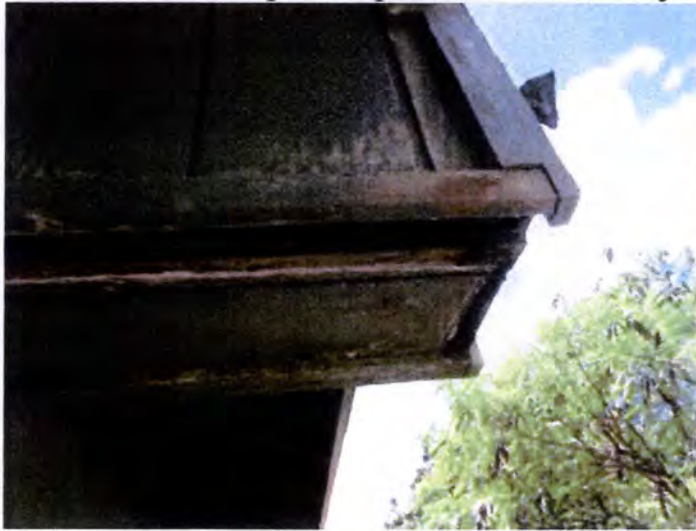
The fascia/soffit areas appeared to be rotted/water damaged/deteriorated at the time of inspection. Recommend having a licensed contractor evaluate and repair/replace as necessary.
