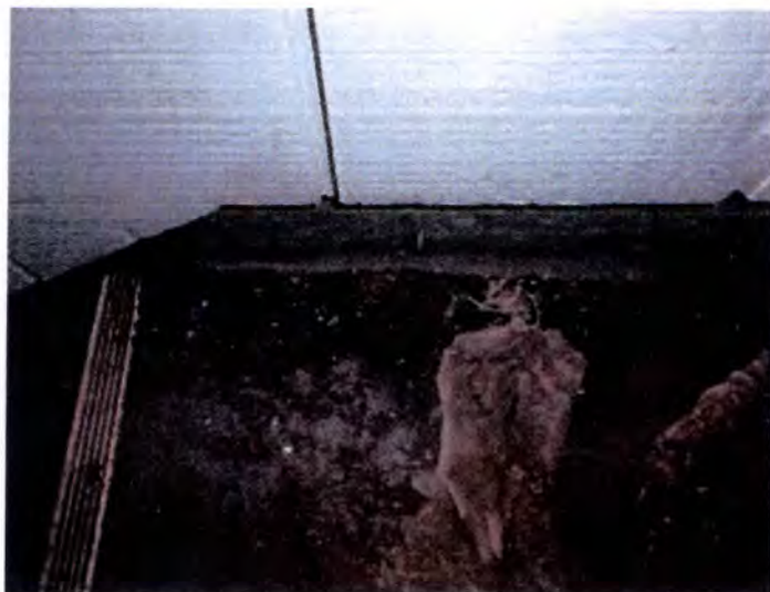
There were visible indications of WDO (Wood Destroying Organism) damage noted at the fascia and soffit areas. Recommend having a licensed contractor evaluate and repair/replace as necessary.
