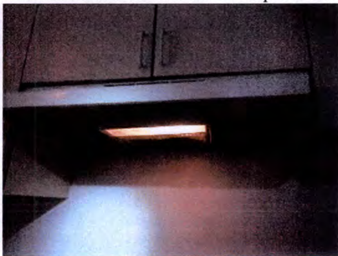
The kitchens in building A appeared to be functional at the time of inspection.
