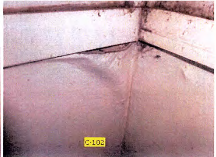
Most of the exterior facing lower interior wall finishes had moisture damage observed. Recommend removal and replacement of affected materials.
