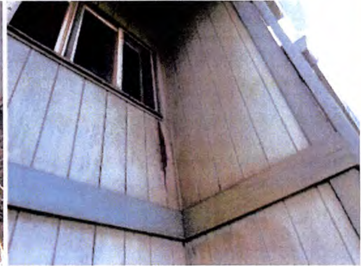
Moisture damage observed at exterior wall areas. Recommend select demolition and replacement of affected ground level exterior siding and finishes.
