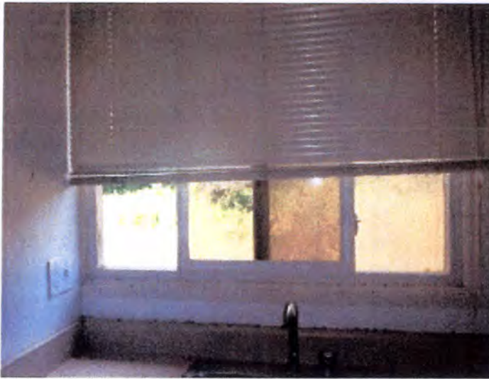
Most of the tested windows operated properly when tested. Except as noted.
