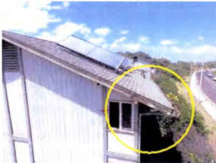
The fascia/soffit areas appeared to be rotted/water damaged/deteriorated at the time of inspection. Recommend having a licensed contractor evaluate and repair/replace as necessary.
