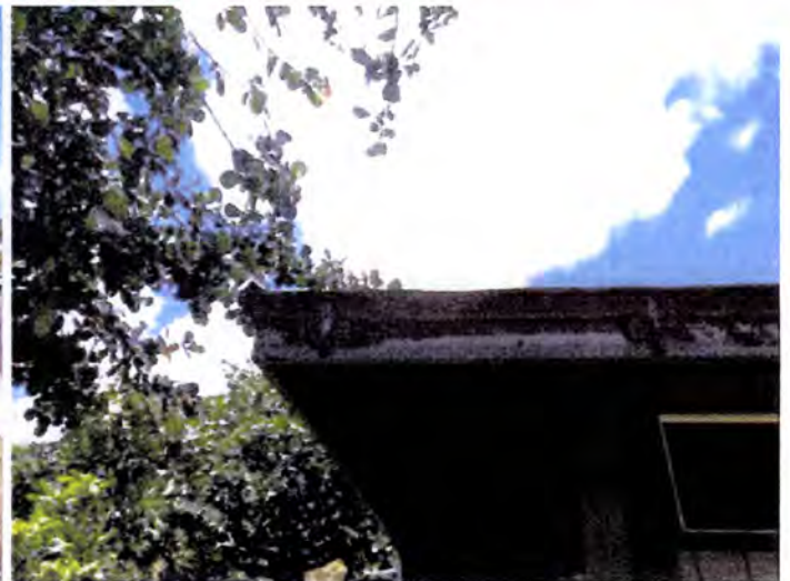
The fascia/soffit areas appeared to be rotted/water damaged/deteriorated at the time of inspection. Recommend having a licensed contractor evaluate and repair/replace as necessary.
