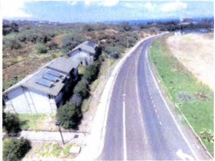
There were no accessibility issues noted at the building.
