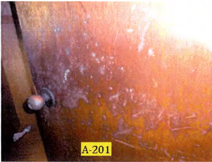
Visible mold observed at interior doors.
