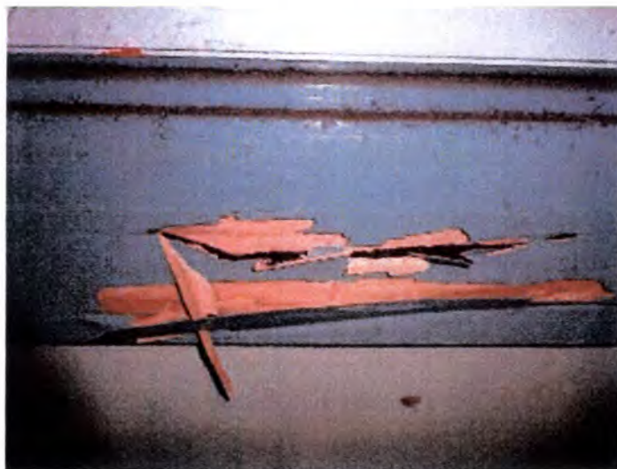
There were visible indications of WDO (Wood Destroying Organism) damage noted at the fascia and soffit areas. Recommend having a licensed contractor evaluate and repair/replace as necessary.
