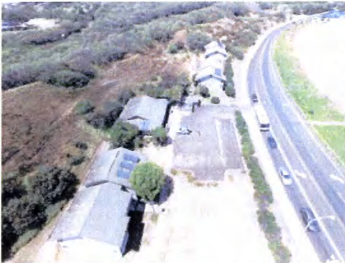
There were no noted obstructions below the 13'-6" minimum.
