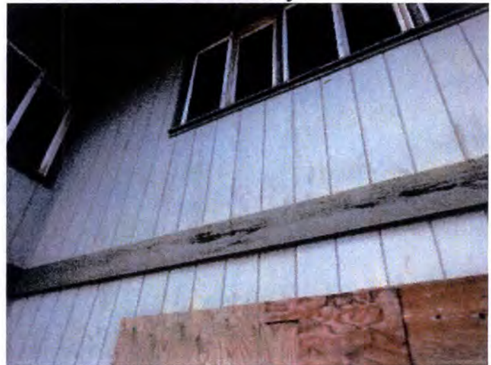
Visible indications of WDO (termite) damage noted. Recommend having a licensed pest contractor evaluate and treat as necessary. Also, recommend having a licensed contractor evaluate and repair/replace damaged material as necessary.
