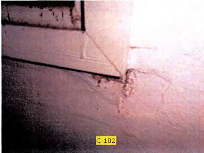
Most of the exterior facing lower interior wall finishes had moisture damage observed. Recommend removal and replacement of affected materials.
