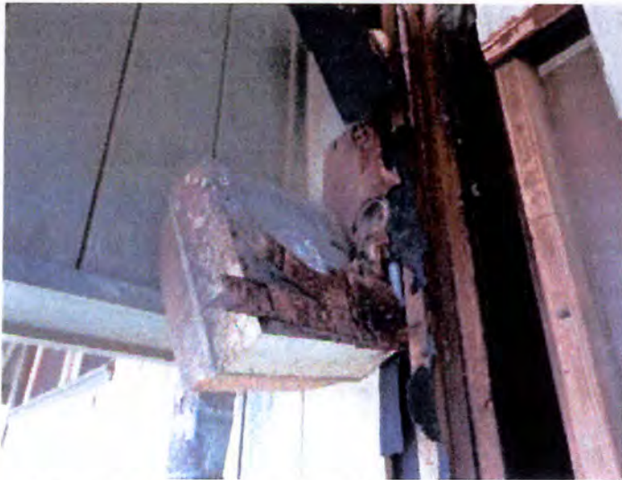
Some of the exterior lighting fixtures were damaged and need to be replaced.
