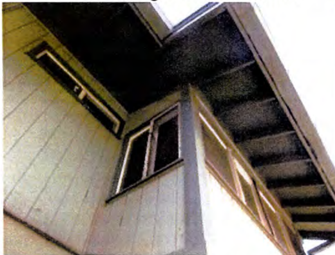
Wood framed wall panels noted
