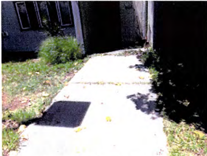
Concrete sidewalks noted.
