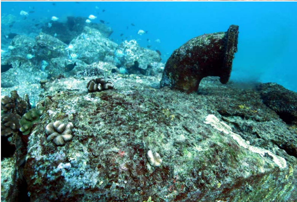
EXHIBIT 1. Photographs of ocean discharge diffusers in Hilo Bay off the Hilo Wastewater Treatment Plant (top) and off Sandy Beach off the East Honolulu Wastewater Treatment Plant (bottom). Both diffusers are at a water depth of approximately 35-40 feet. Concentrated streams of treated effluent of high nutrient concentration, low salinity, and elevated temperature relative to receiving water can be clearly seen in both photos. Note presence of live corals on both outfall structures, lack of presence of filamentous algae, and clarity of water. Both ocean outfalls have been in operation since the 1970's. All photographs taken by S. Dollar in 2014.
