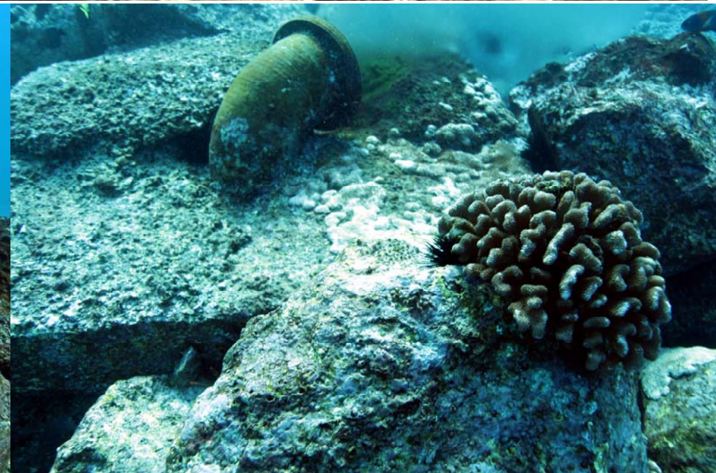
EXHIBIT 1. Photographs of ocean discharge diffusers in Hilo Bay off the Hilo Wastewater Treatment Plant (top) and off Sandy Beach off the East Honolulu Wastewater Treatment Plant (bottom). Both diffusers are at a water depth of approximately 35-40 feet. Concentrated streams of treated effluent of high nutrient concentration, low salinity, and elevated temperature relative to receiving water can be clearly seen in both photos. Note presence of live corals on both outfall structures, lack of presence of filamentous algae, and clarity of water. Both ocean outfalls have been in operation since the 1970's. All photographs taken by S. Dollar in 2014.
