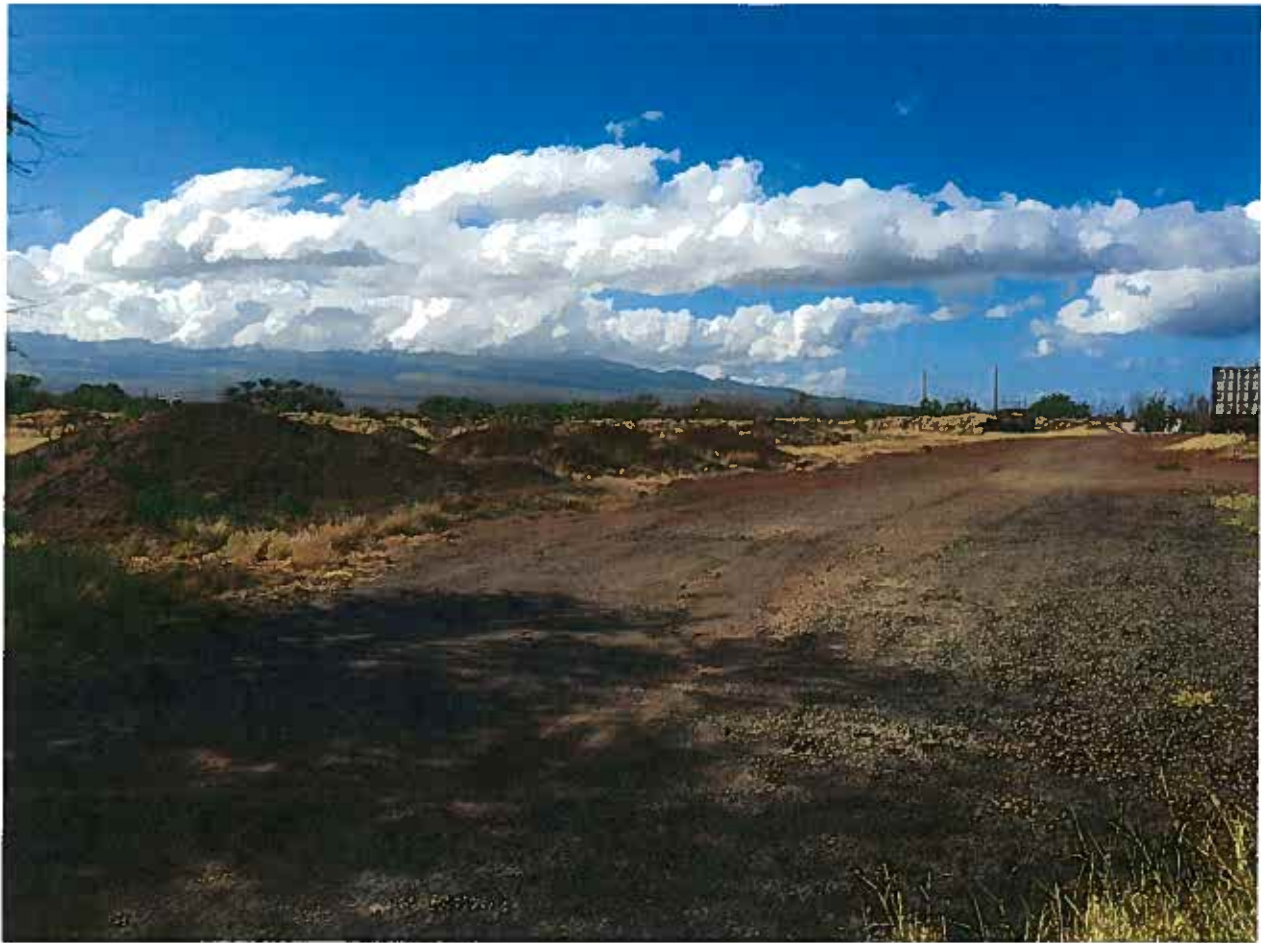
Figure 8. Base yard truck road, gravel and top soil piles.
