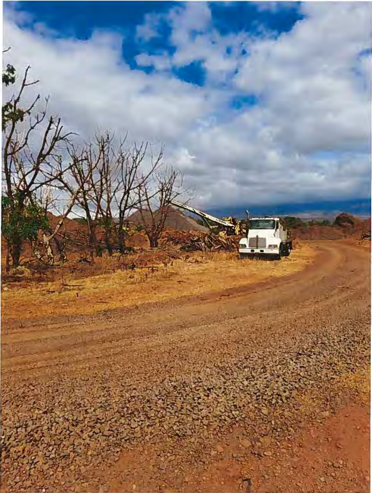
Figure 13: Overview of property from Southwest corner, view to Northeast
