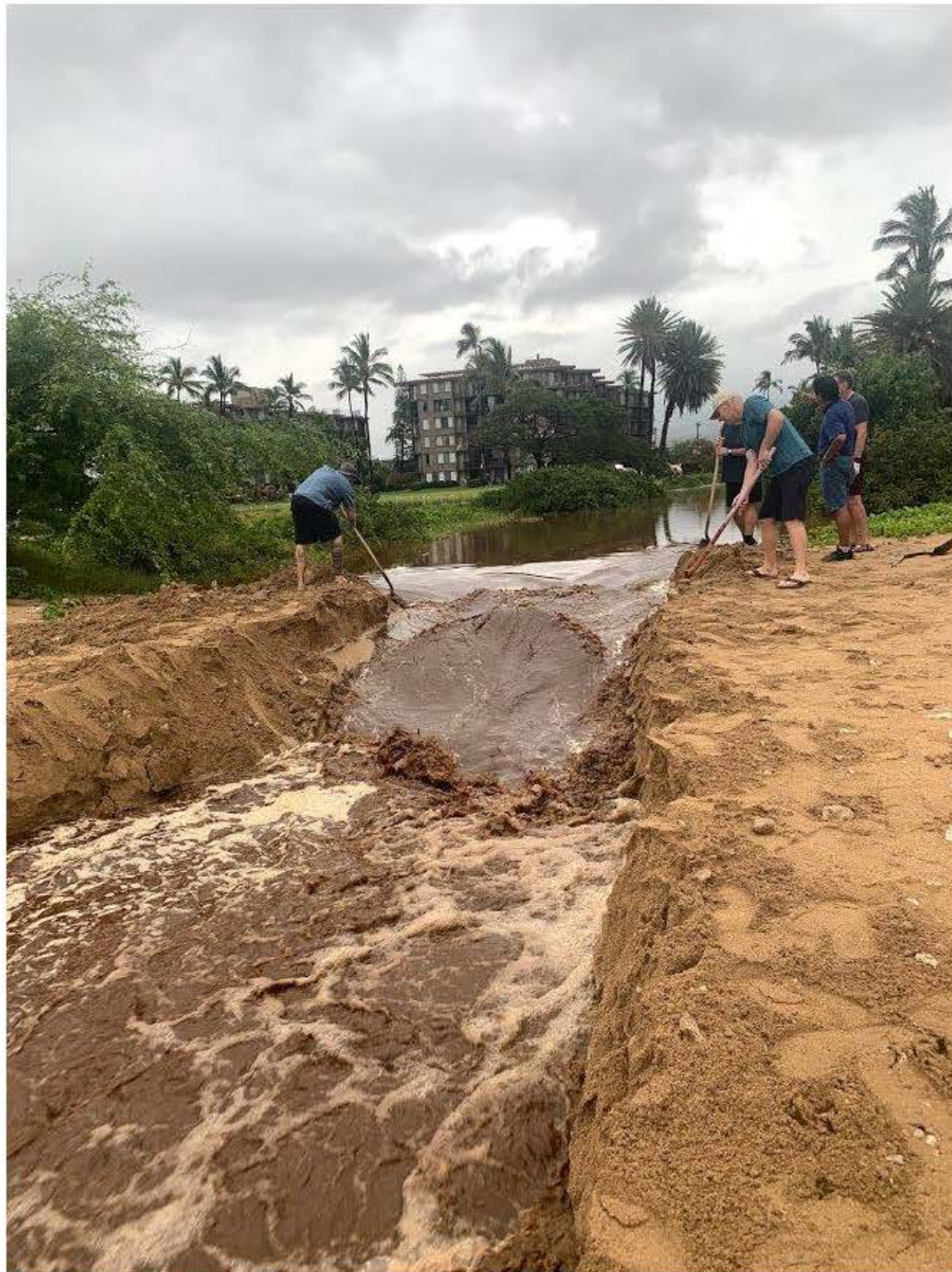
Waipuilani Wetland Stream - Dune Breaking
