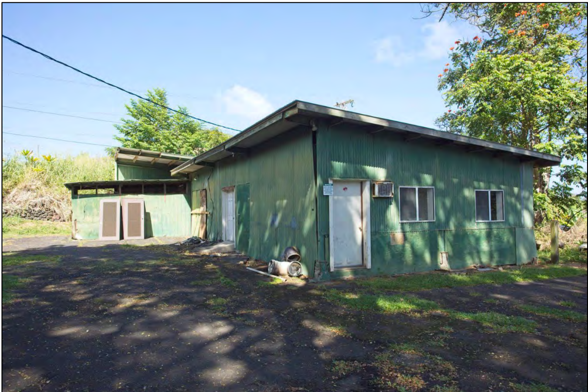
Photo 10, Wooden storage building from
