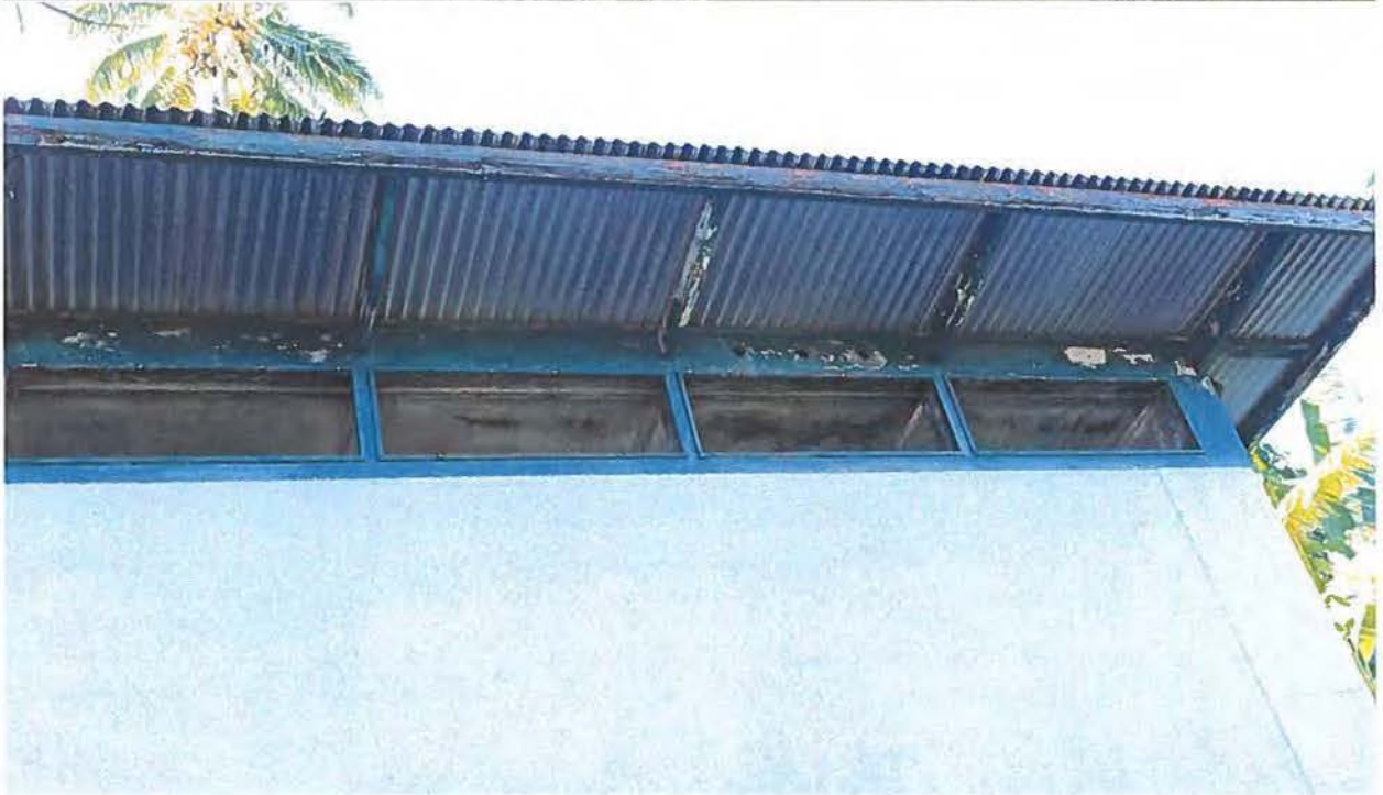
Figure 2 - Clerestory openings on 20th century addition.
