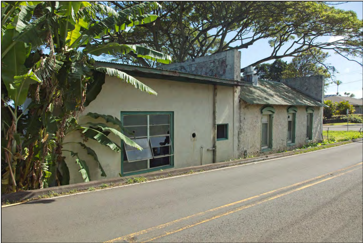
Photo 3, Side of historic storage building and later addition from Hana Highway looking East
