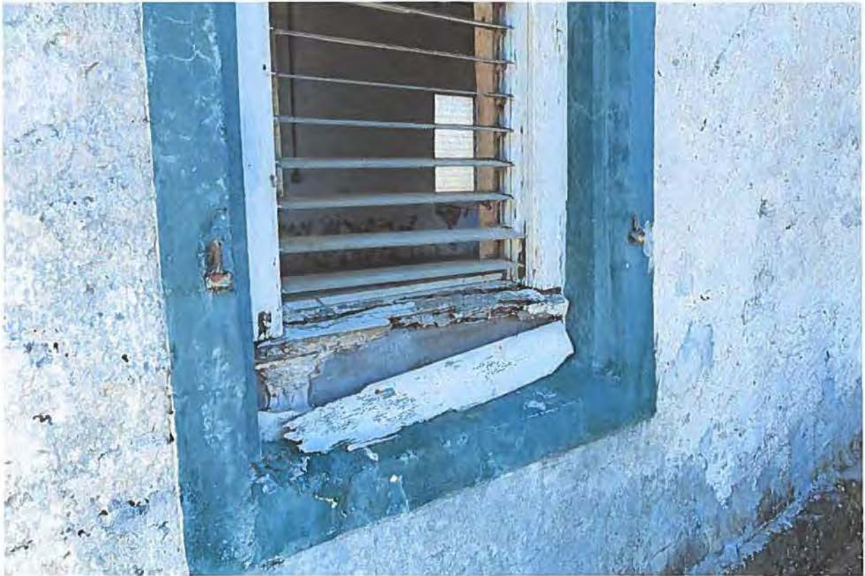
Figure 1 - Shutter hinges visible on historic window surrounds.
