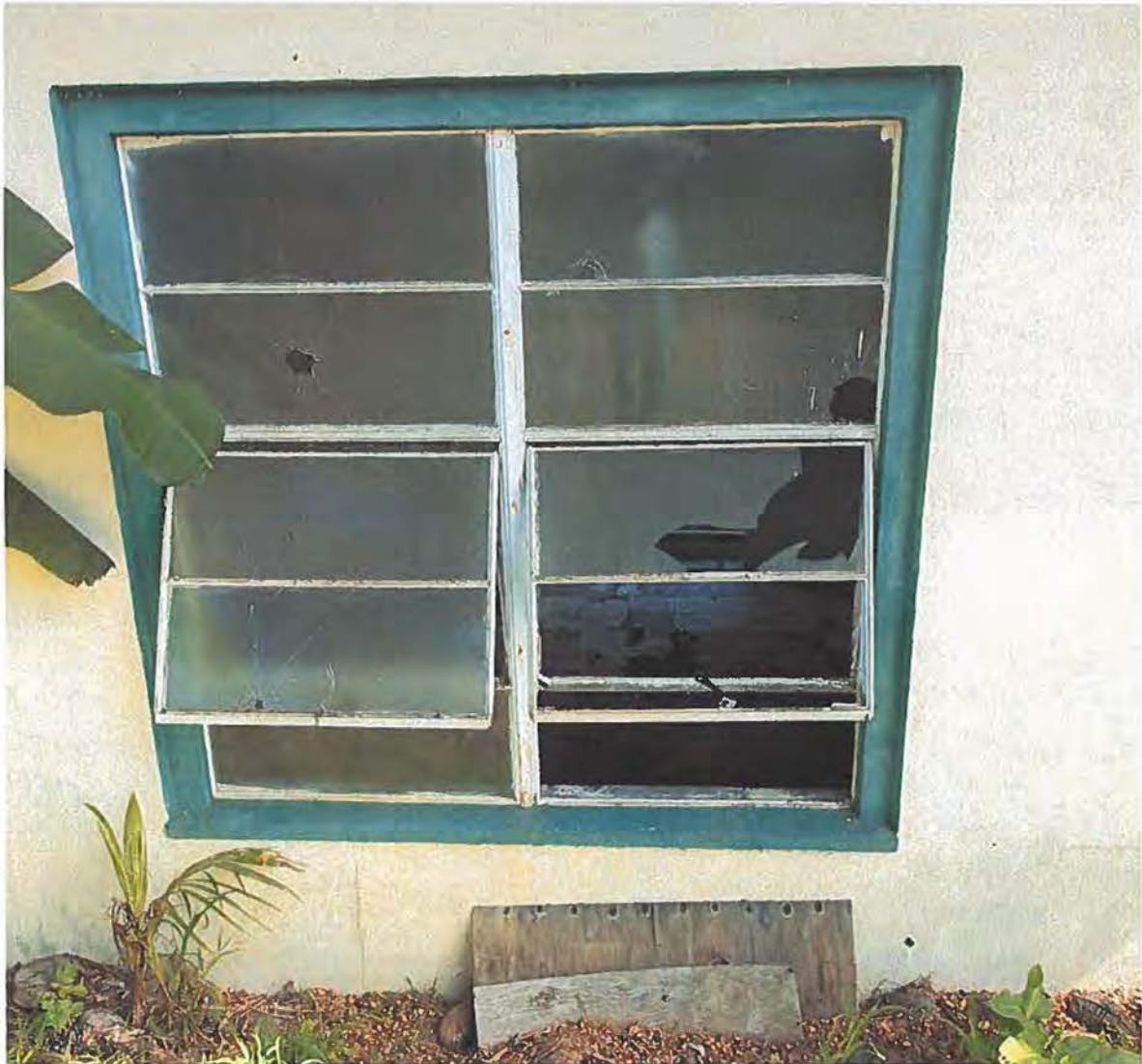
Figure 3 - Metal-framed awning windows on 20th century addition.
