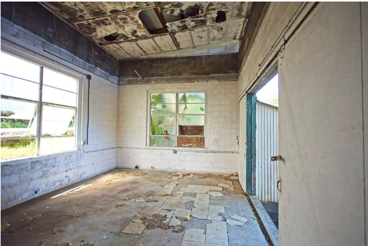
Photo 8, Interior of addition
