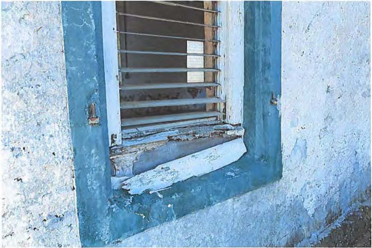
Figure 1 - Shutter hinges visible on historic window surrounds.
