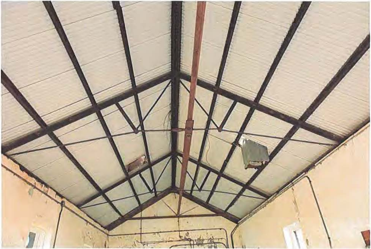
Figure 5 - Interior roof framing in original portion of the building.
