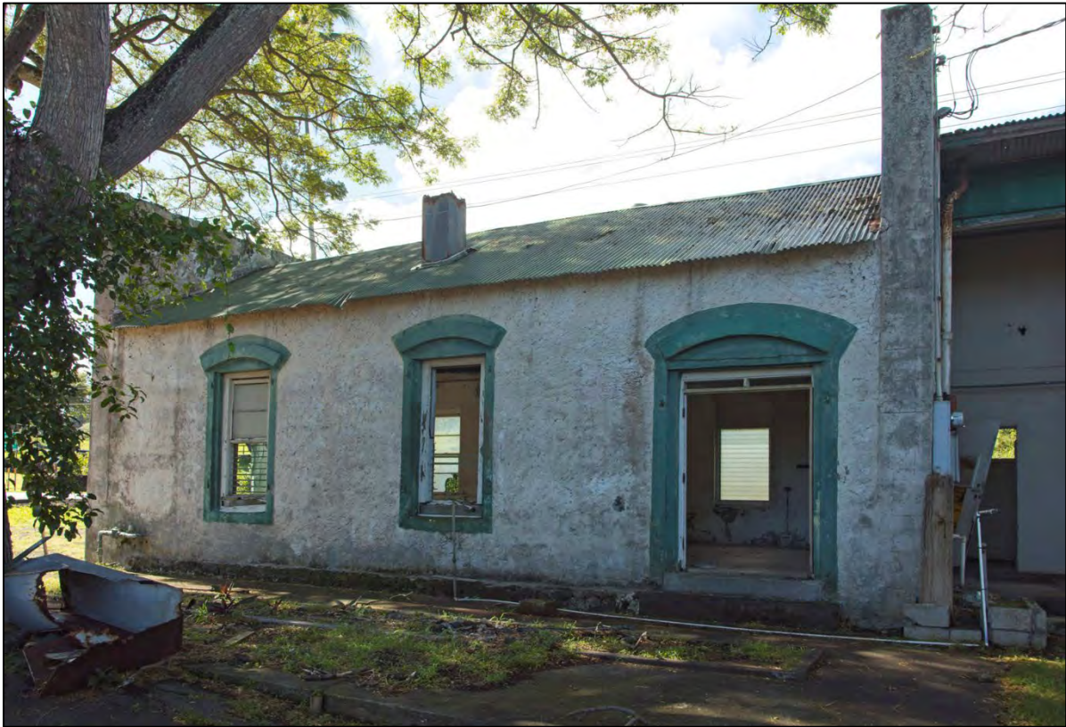
Photo 5, Historic storage building from on the property looking West
