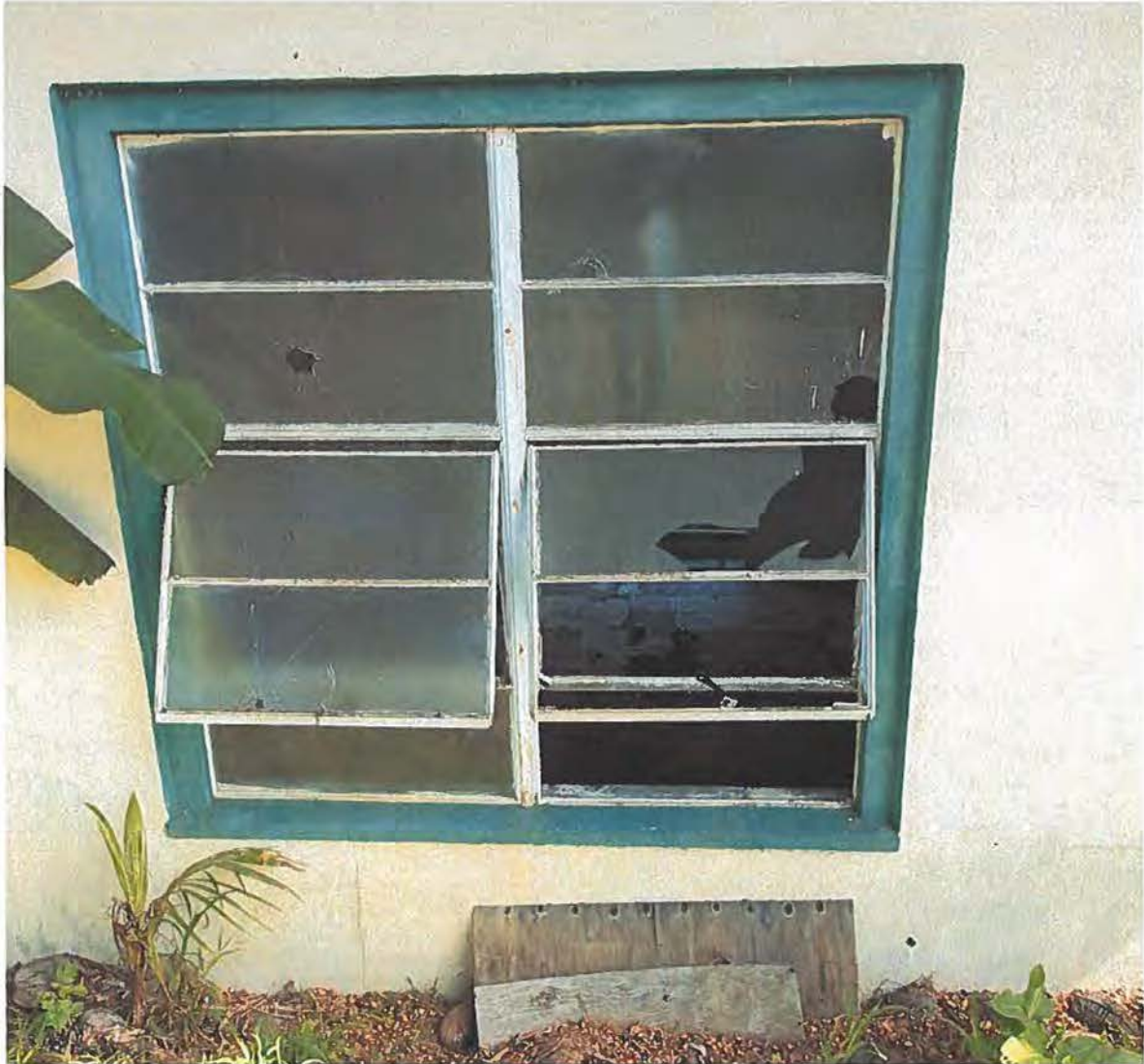
Figure 3 - Metal-framed awning windows on 20th century addition.
