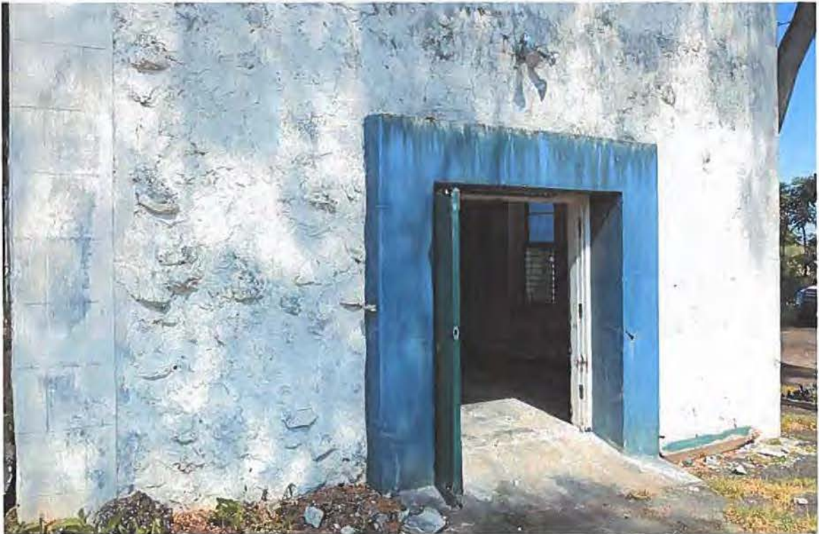
Figure 4 - Photo demonstrating unique texture of the historic masonry walls.
