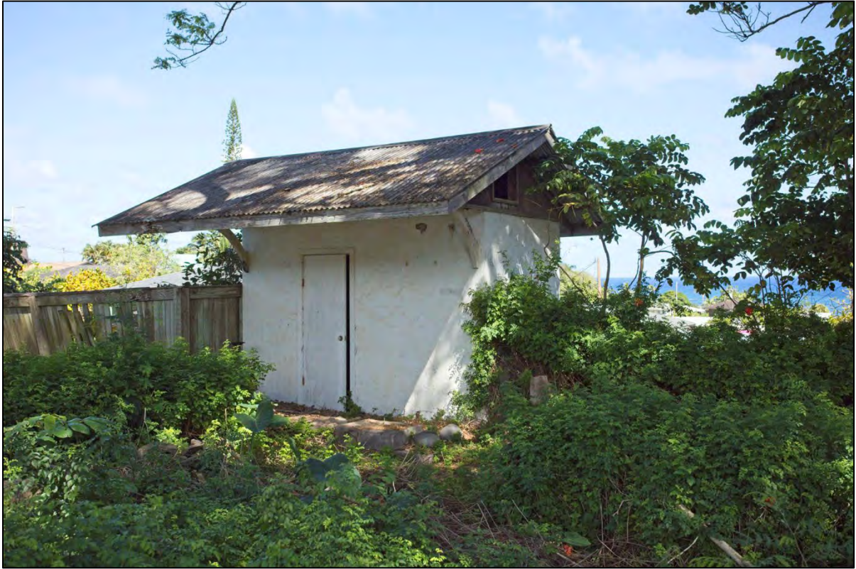
Photo 11, Old storage shed looking East
