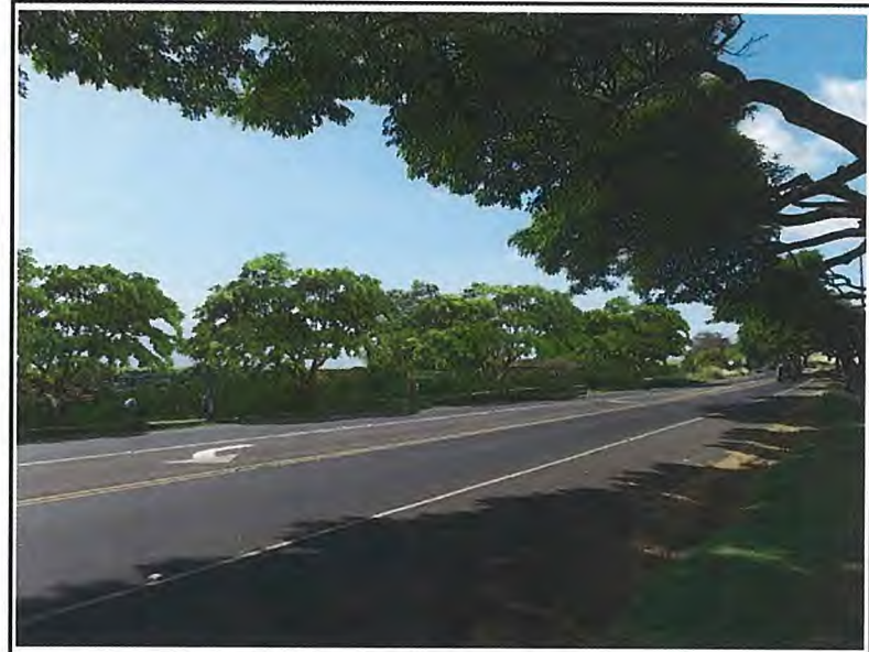
2. After. Looking in a south-easterly direction over the makai development with canopy trees in the background and separated pedestrian and bicycle path in the foreground.
