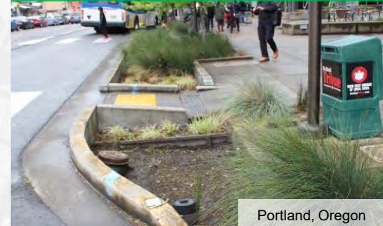
Rain Garden Curb Extensions
