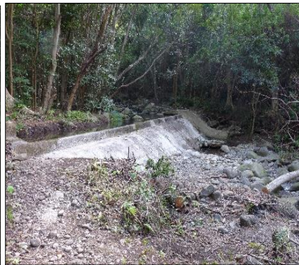
Figure 28: S. Waikapū Dam Intake Diversion (2012)
