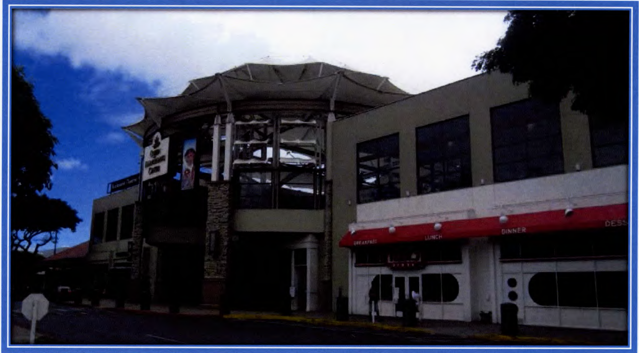
Commercial Shopping Center on Industrial Zoned Land – Industrial Classification
