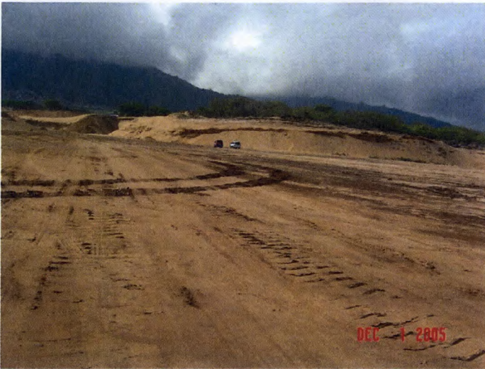
AMERON SAND EXCAVATION SITE AT MAUI LANI
